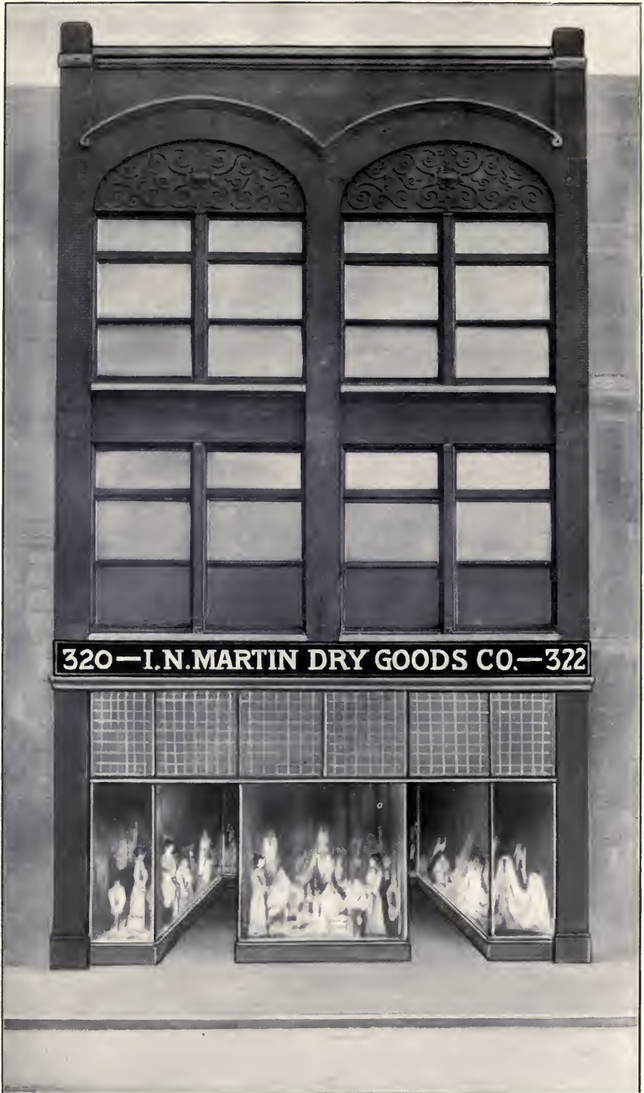
The New Home of the I. N. Martin Dry Goods Co., 320-322 South Adams Street
