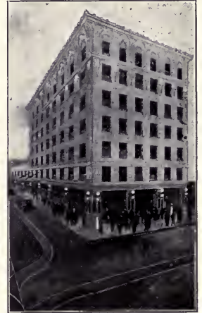
Illinois Traction System Bldg. now under construction.
