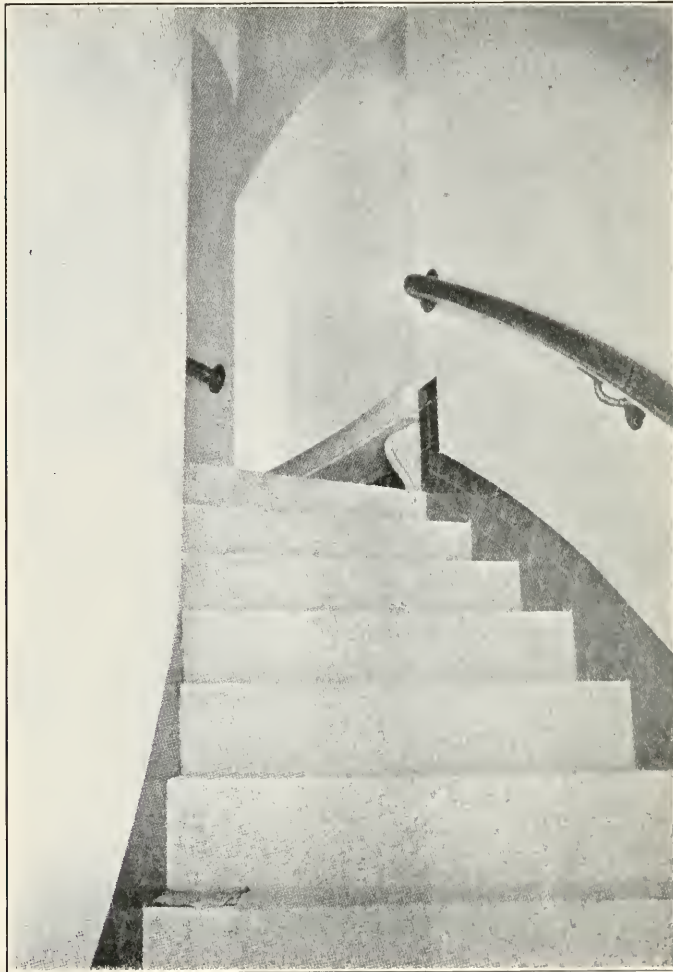
ASCENDING TO THE ELEVATOR FLOOR
