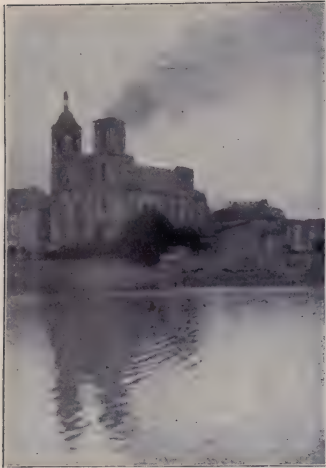
BURNING CHURCH AT PONT-À-MOUSSON STRUCK BY INCENDIARY SHELL
