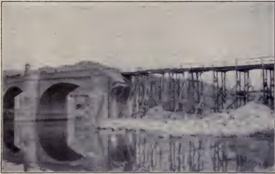
BRIDGE OVER MOSELLE AT PONT-À-MOUSSON
