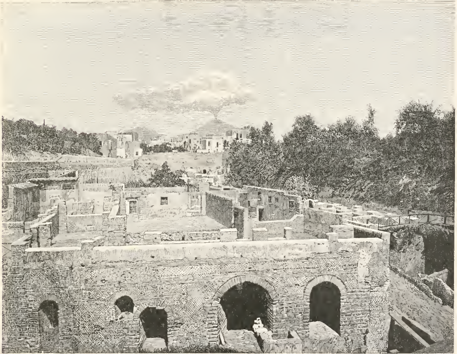
VIEW OF EXCAVATED PORTION OF POMPEII, LOOKING NORTHWEST.
