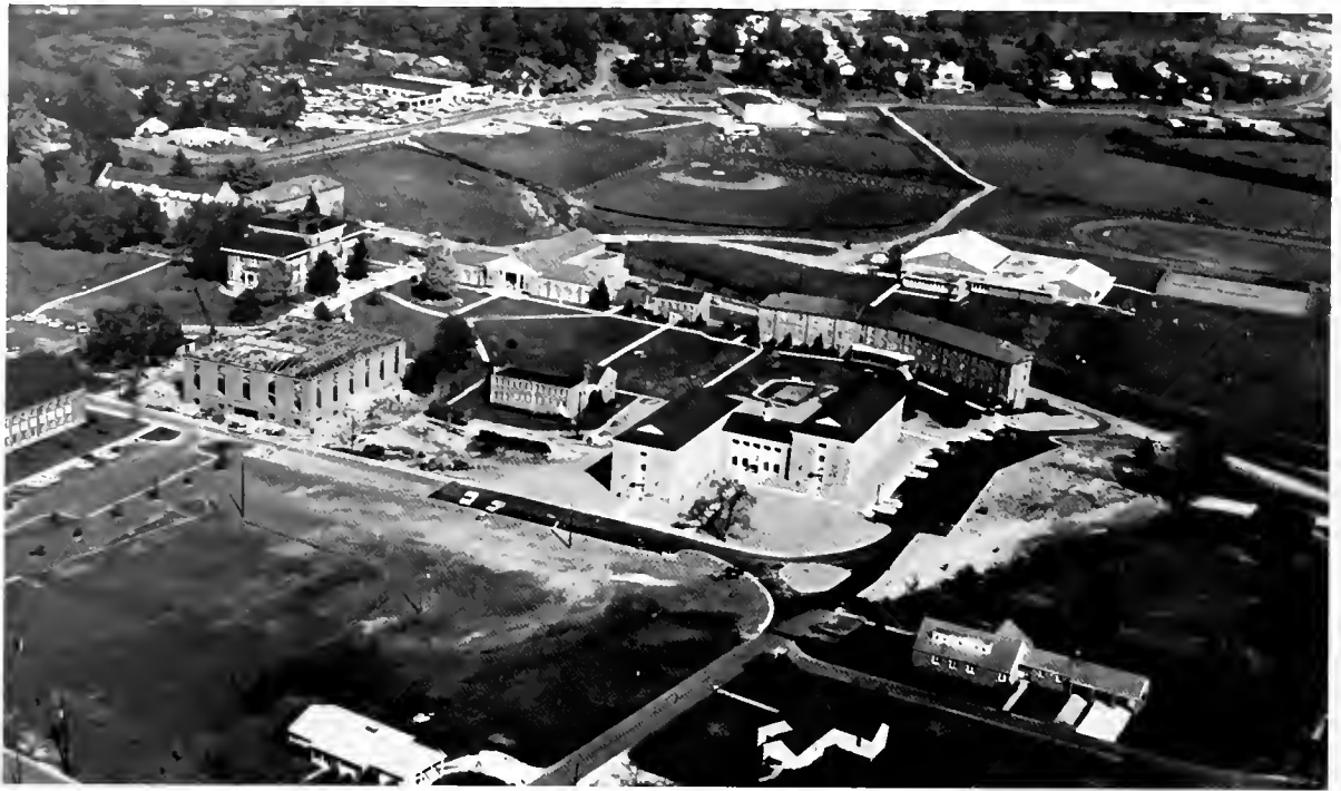
AERIAL VIEW, BREVARD COLLEGE CAMPUS
