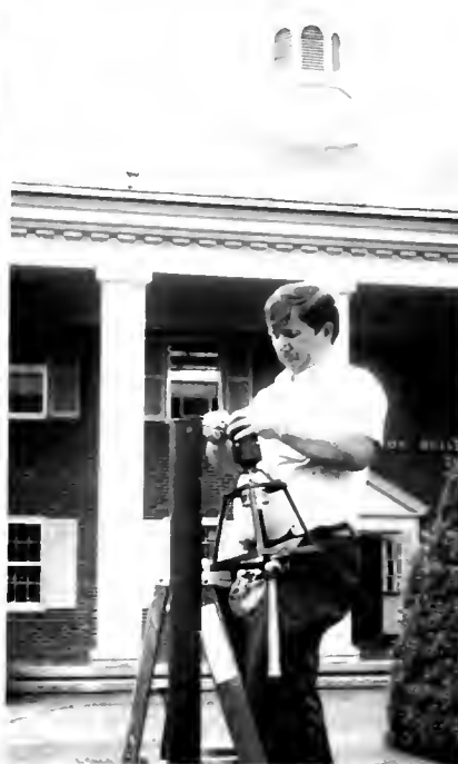
Gary works hard to repair the light so the students are able to see at night.
