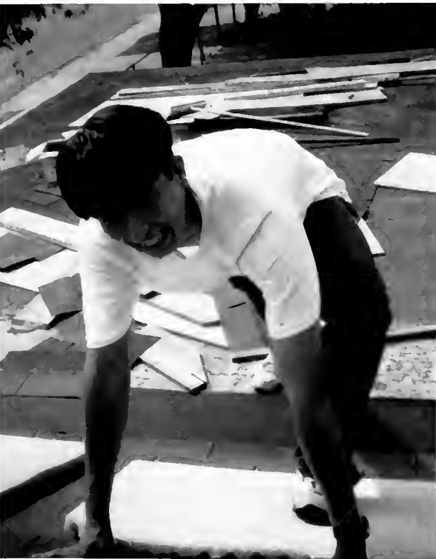
Hiromi Yamada assists in reroofing a home in Brownsville, Texas.
