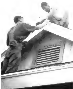
Brad Dodson and Toshi Akita repair a roof in Brownsville, Texas.
