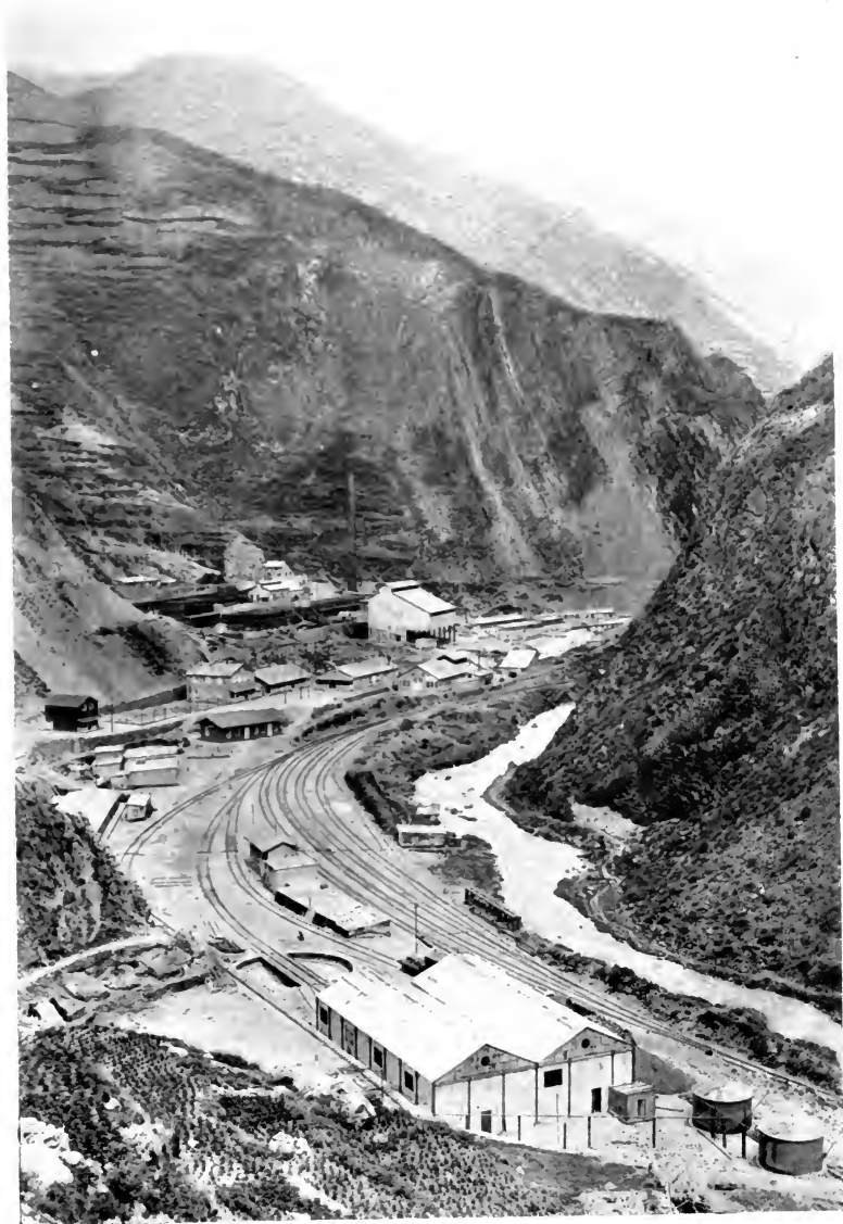
RIO BLANCO, SHOWING RAILWAY STATION (SOUTHERN RAILWAY COMPANY) AND SMELTER.
