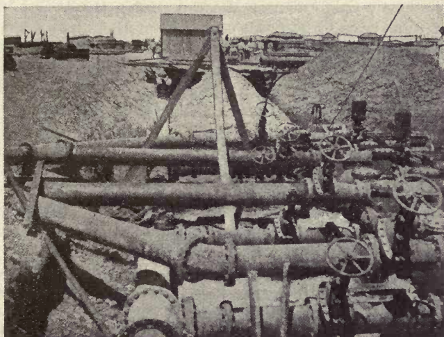
OIL PIPE-LINE CONNECTIONS IN THE AMERICAN FIELDS
