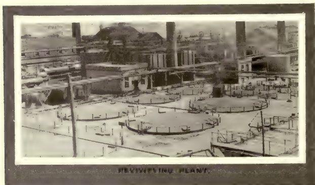
Copper Sulphide is here purified so that it may be used again.
