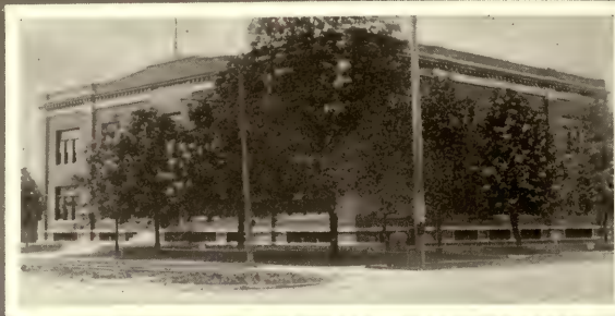
REFINERY OFFICE, BARNIA
