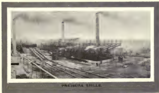
For obtaining additional yield of Gasoline by Burton process.
