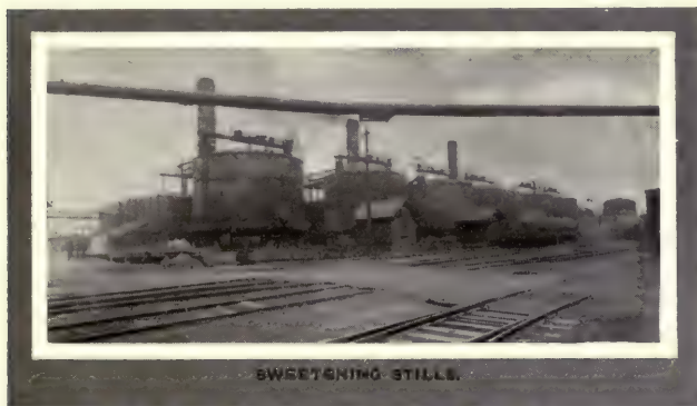
Oils are here freed of sulphur by copper oxide.
