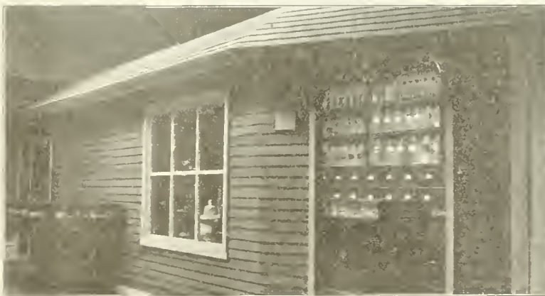
Exterior of the Old Store
