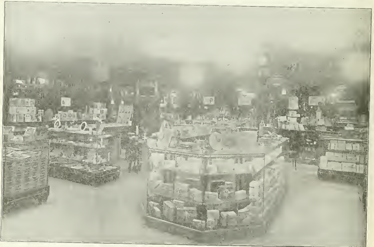
Fig. 5—A Well Lighted Drug Store Using Mazda Lamps and Semi-Indirect Reflectors. You Will Note the Evenness of Illumination and Absence of Shadows.
