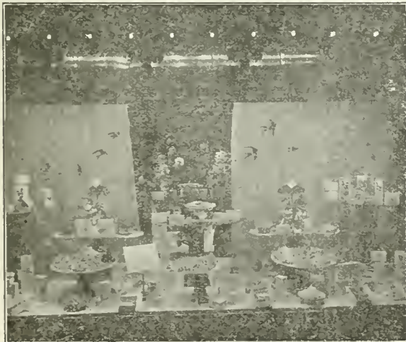
Fig. 7—A Well Lighted Window Using Mazda Lamps with Mirrored Glass Reflectors Located at the Front Upper Edge of the Window.
