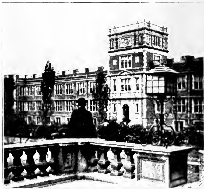
Medical Building From the Dormitory Terrace
