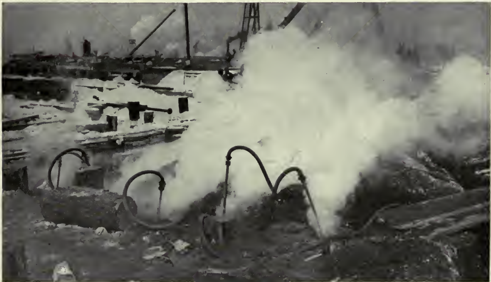
Thawing Ground at Hog Island with live steam.
