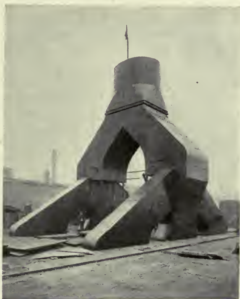
Uptake and Base for 7,500 D. W. Ton Freight Carrier.
