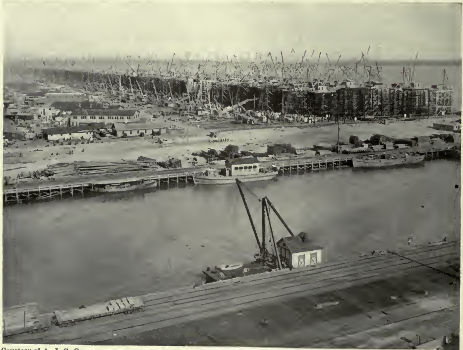
Shipways at Hog Island, East from Bridge Crane.
