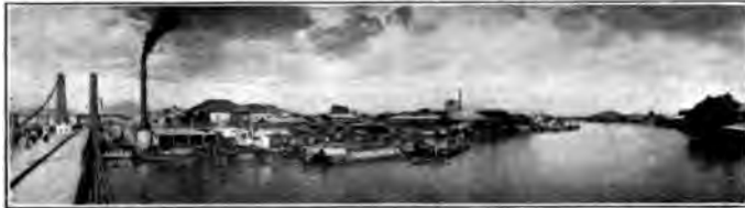
SUSPENSION BRIDGE OVER PASIG RIVER
