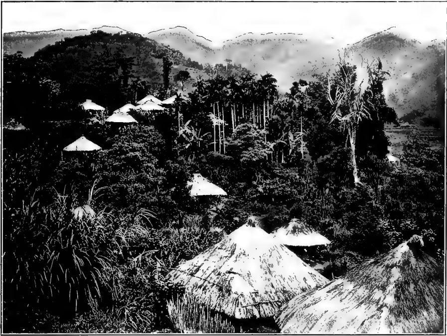
FIG. 2. IFUGAO SETTLEMENT, PART OF QUIANGAN.
