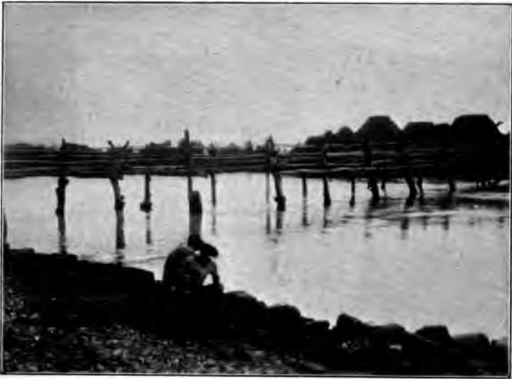
A TYPICAL OLD-STYLE BRIDGE.
