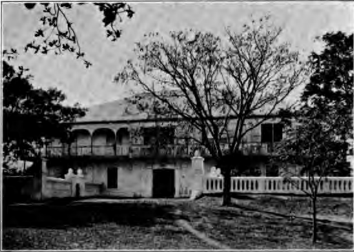
A TYPICAL OLD-STYLE PROVINCIAL GOVERNMENT BUILDING.
