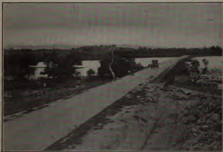
NEW-STYLE ROAD ACROSS LOWLANDS.
