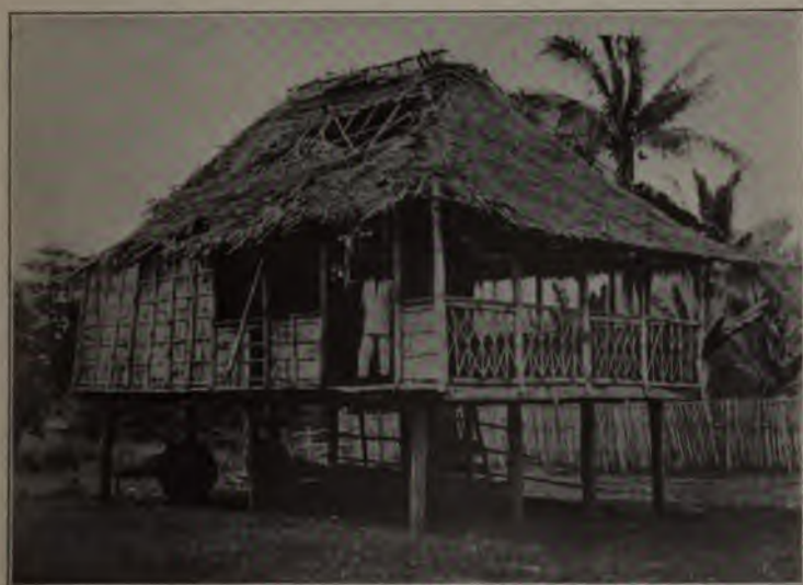
A TYPICAL NEGLECTED FILIPINO HOUSE.
