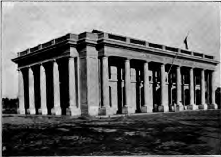
A MODERN PROVINCIAL GOVERNMENT BUILDING.
