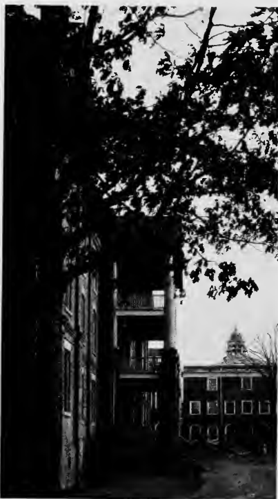
WEST DORMITORY (Front View)
