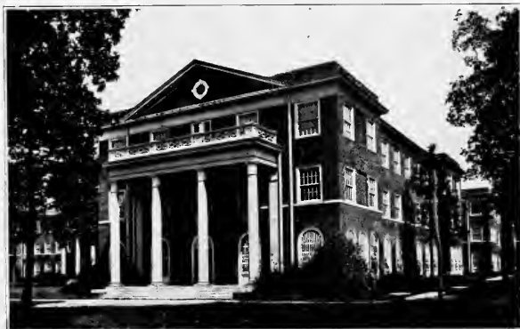
One of the five new and modern administrative buildings on the Elon Campus
