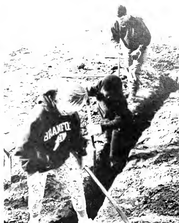
Students work in a ditch to help housing cause
