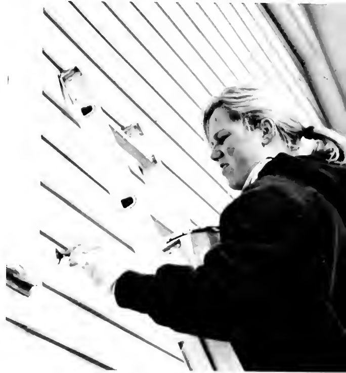
Kati Mafko puts the finishing touches on a window ledge
