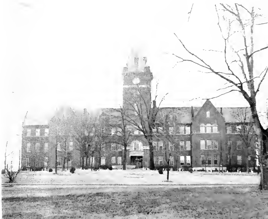
FRONT VIEW MEMORIAL HALL
