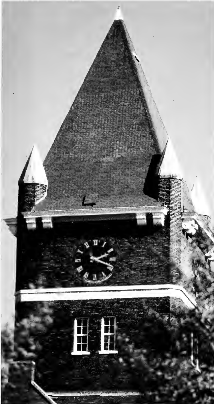
Cumberland University's Memorial Hall is the focal point of the campus. As Lebanon, Tennessee's tallest landmark, the distinctive clock tower can be seen from all over the city.
