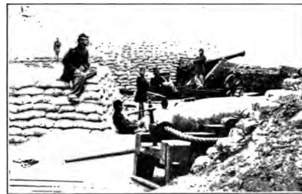
GUNS THE UNION LOST AND RECOVERED. (A two-gun Confederate battery in the entrenchments south of Yorktown.) The near gun is a 32-pounder Navy gun which had been burst, wrecking its embrasure. The far one, a 24-pounder siege-piece. More than 3,000 pieces of naval ordnance fell into the hands of the Confederates early in the war, through the ill-advised and hasty abandonment of Norfolk Navy Yard by the Federals. Many of these guns did service at Yorktown and subsequently on the James River against the Union.
