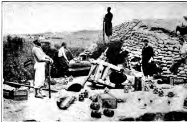
WRECKED ORDNANCE. (Gun exploded by the Confederates on General Hill's rampart, Yorktown.) Although the Confederates abandoned 200 pieces of ordnance at Yorktown, they were able to render most of them useless before leaving. Hill succeeded in terrorizing the Federals with grape-shot, and some of this was left behind. After the evacuation the ramparts were overrun by Union trophy seekers. The soldier resting his hands upon his musket is one of the Zouaves whose bright and novel uniforms were so conspicuous early in the war. This spot was directly on the line of the British fortification of 1781.
