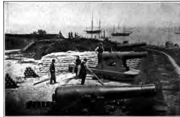
THE CONFEDERATE COMMAND OF THE RIVER. (Battery Magruder, Yorktown.) Looking north up the river, four of the five 8-inch Columbiads composing this section of the battery are visible. The grape-shot and spherical shells, which had been gathered in quantities to prevent the Federal fleet from passing up the river, were abandoned on the hasty retreat of the Confederates, the guns being spiked. The vessels in the river are transport ships, with the exception of the frigate just off shore.
