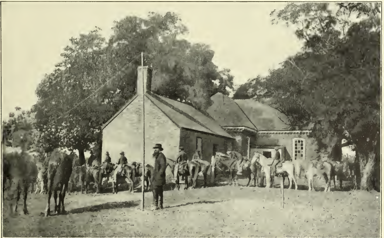
CHARLES CITY COURT HOUSE, VIRGINIA, JULY, 1862
