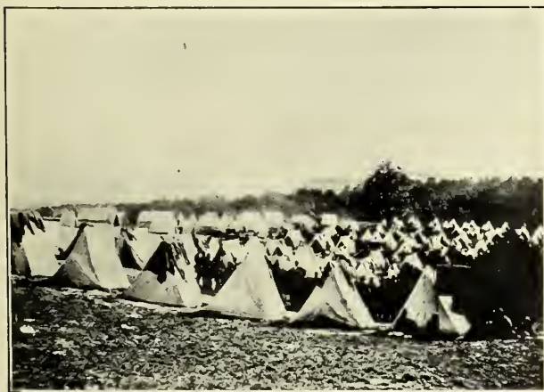
THE CITY OF TENTS. The Army of the Potomac encamped in readiness for the forward movement on Richmond. These comfortable canvas houses were transported by the army wagons. The Confederates had no such complete shelter during the spring of 1862, which was remarkable for the inclemency of the weather.
