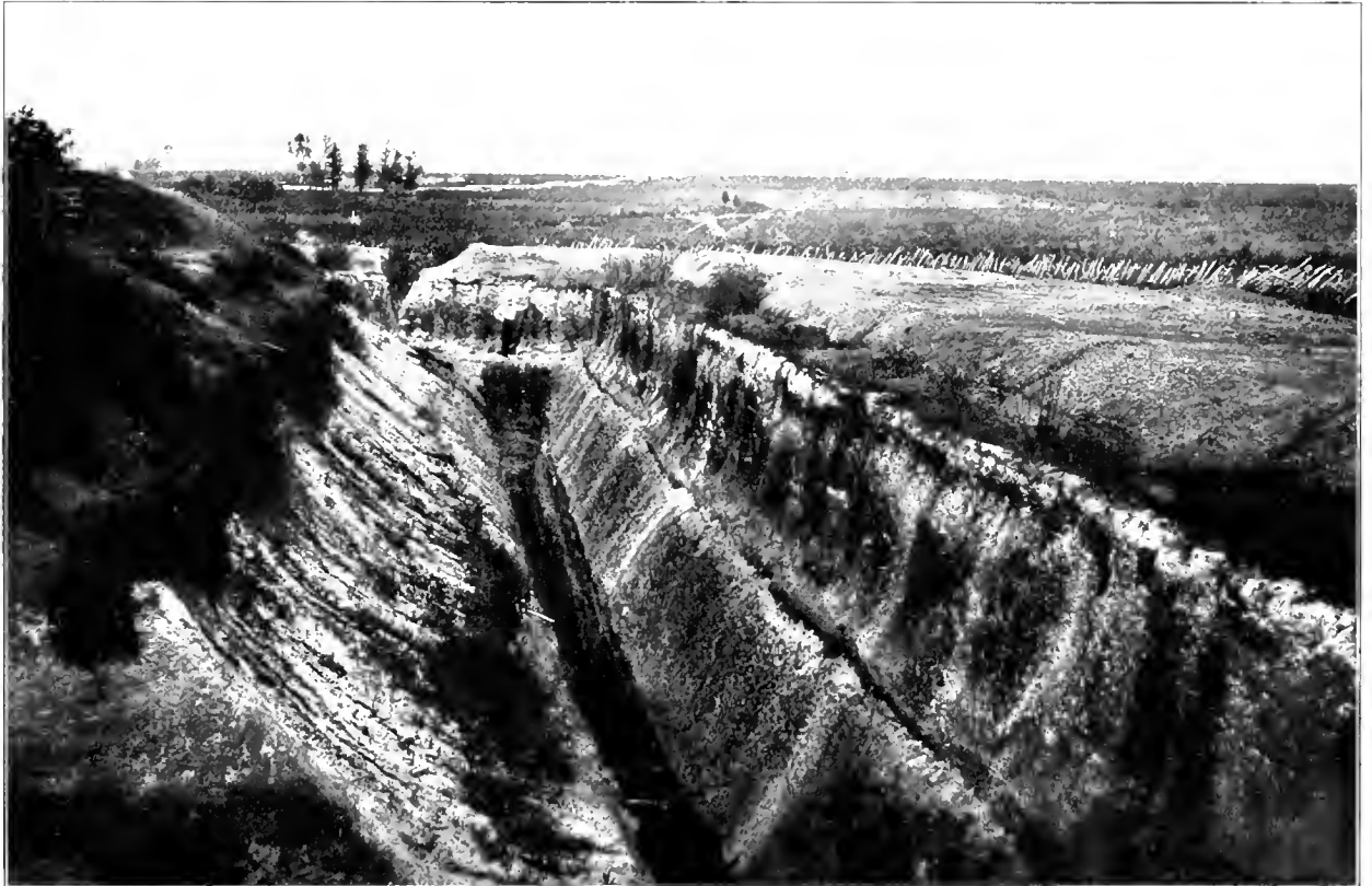
THE 27-FOOT DITCH AT FORT GILMER, GUARD AGAINST FEDERAL MINES
