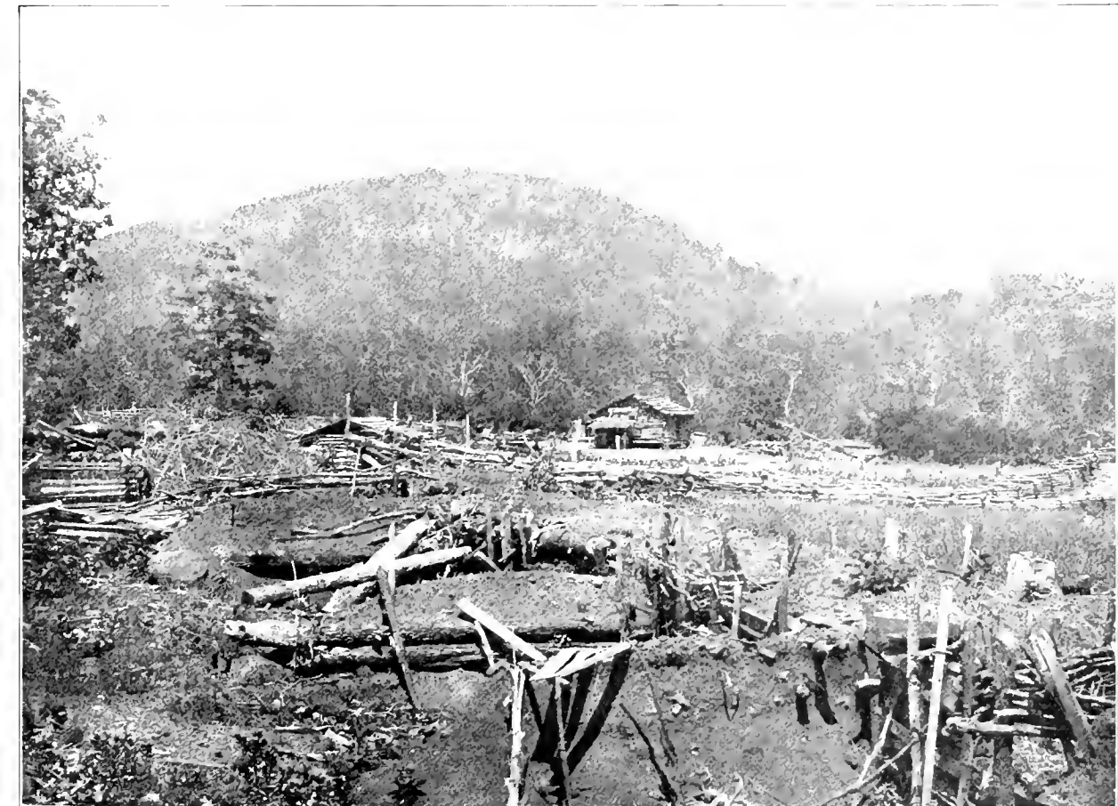
FEDERAL ENTRENCHMENTS AT THE FOOT OF KENESAW MOUNTAIN
