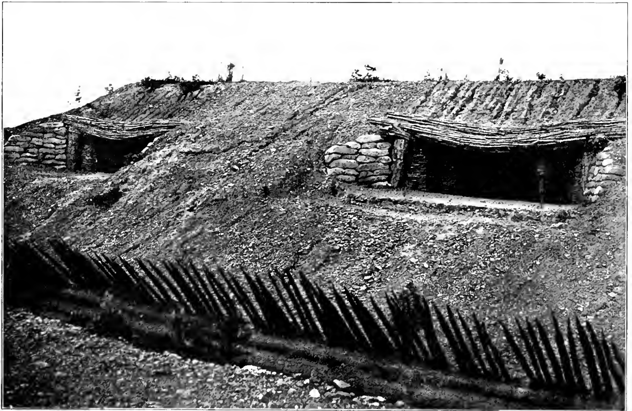
PALISADES AND PARAPET AT FORT HARRISON
