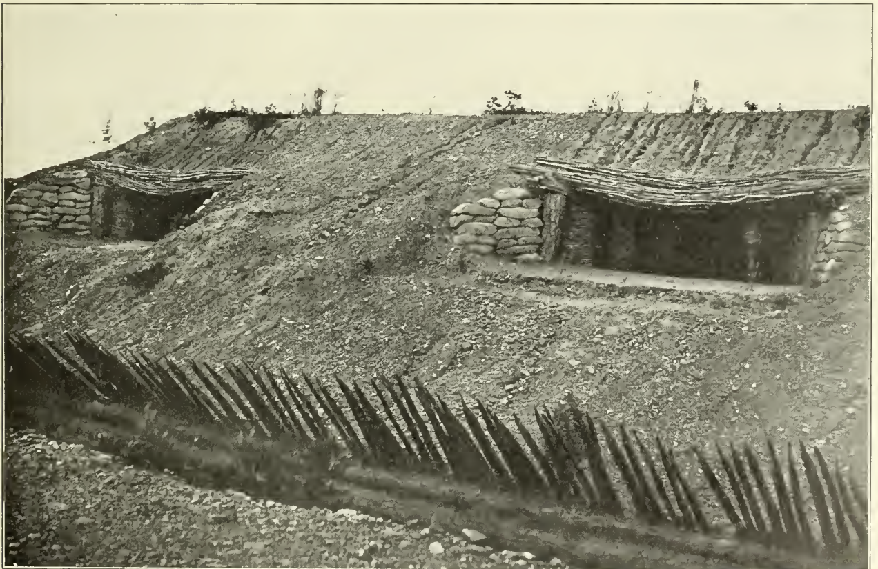
PALISADES AND PARAPET AT FORT HARRISON
