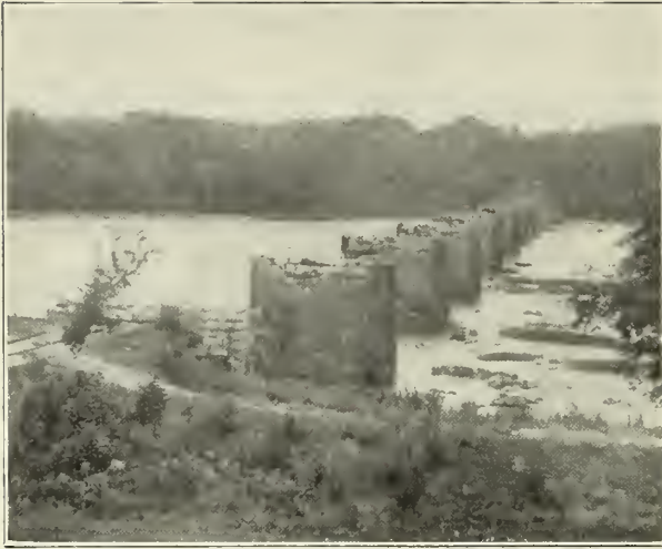
THE CONGAREE RIVER BRIDGE
