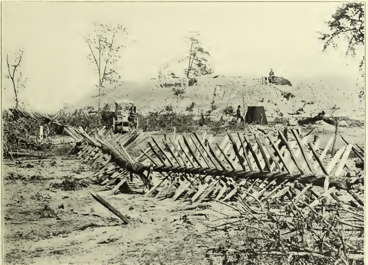
A CLOSER VIEW OF THE ENTANGLEMENTS ON MARIETTA STREET—CHEVAUX-DE-FRISE
