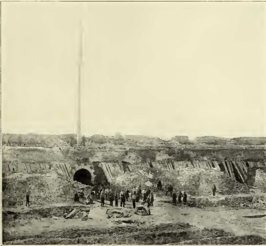
A "COVERED WAY" IN FORT PULASKI, APRIL, 1862—THE GARRISON HERE MADE A CONTINUOUS BOMB-PROOF BY LEANING TIMBERS AGAINST THE INNER WALL OF THE FORT AND THEN COVERING THEM WITH EARTH
