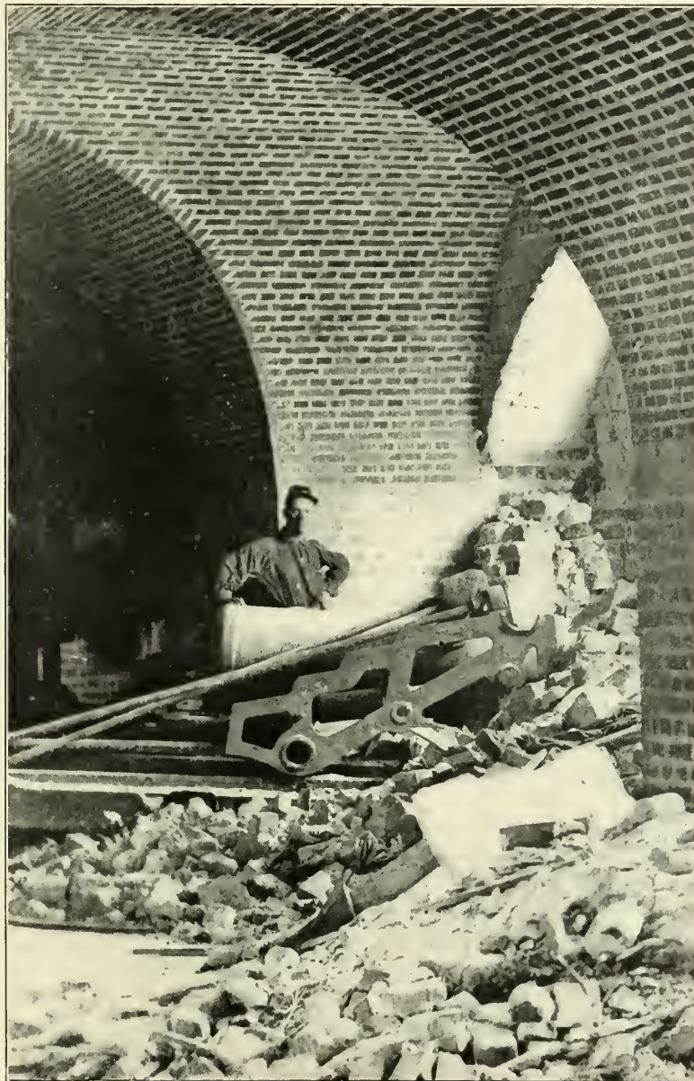
INSIDE THE BREACHED CASEMATE (SEE ABOVE)
