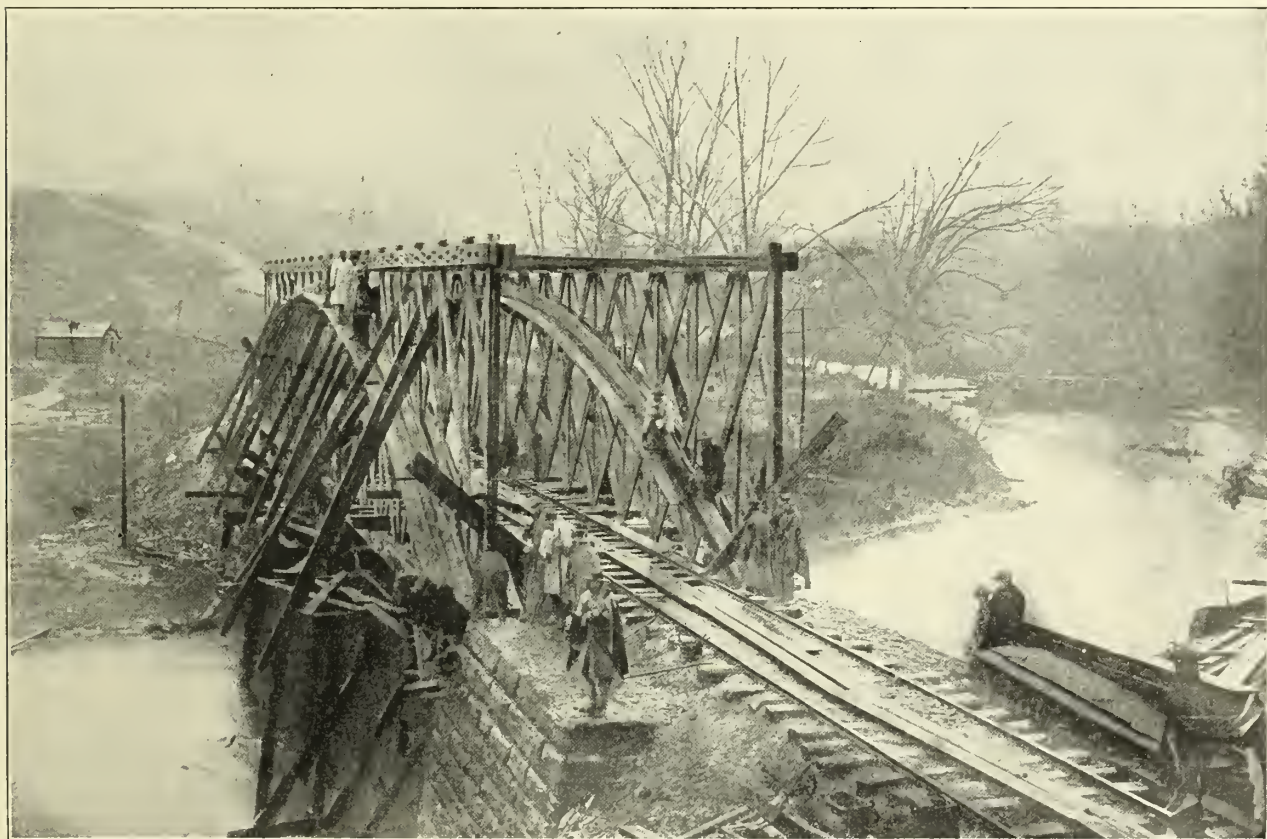
REINFORCED WITH TRUSSES—TRANSFORMED INTO A STANDARD BRIDGE
