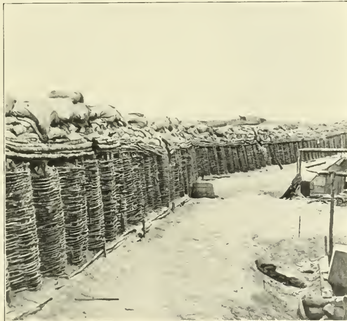
SEDGWICK—GABIONS HEIGHTENED BY SAND-BAGS
