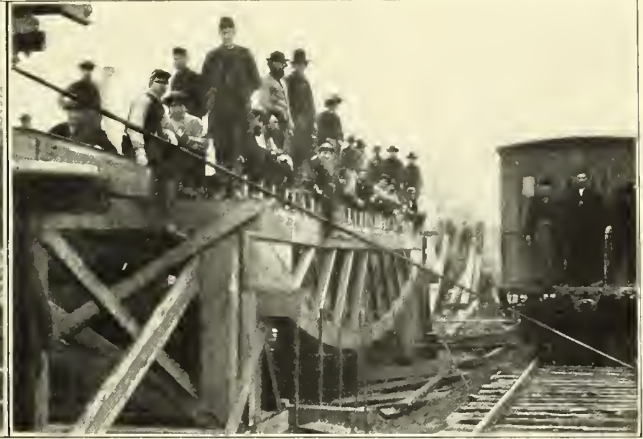
LOADING A BRIDGE TO TEST IT
