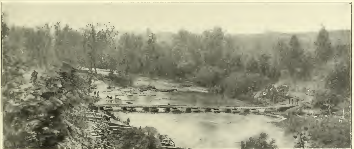
THE BRIDGE FROM UPSTREAM, JERICO MILLS
