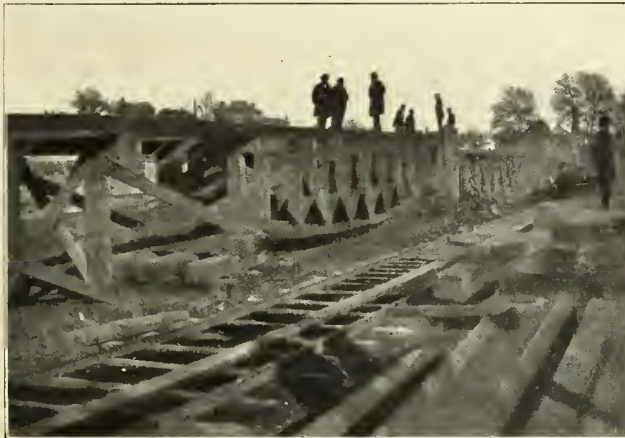
TESTING A "SHAD-BELLY" BRIDGE
