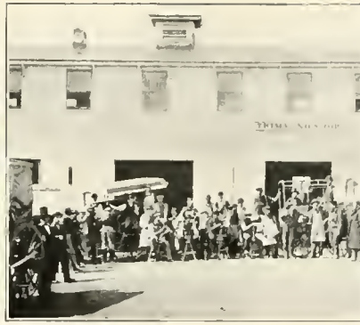
GOVERNMENT TRIMMING SHOP
