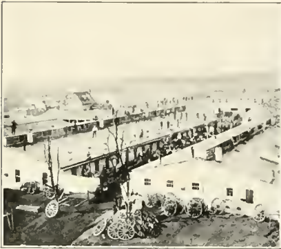
OUTSIDE THE REPAIR SHOPS
