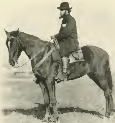
WAUD AT HEADQUARTERS, 1864,
