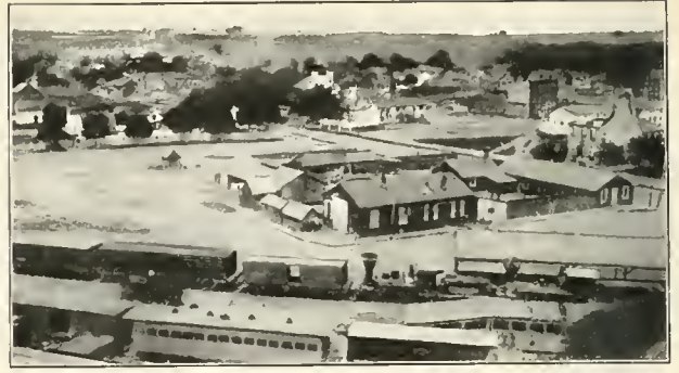
COMMISSARY BUILDINGS AT ALEXANDRIA
