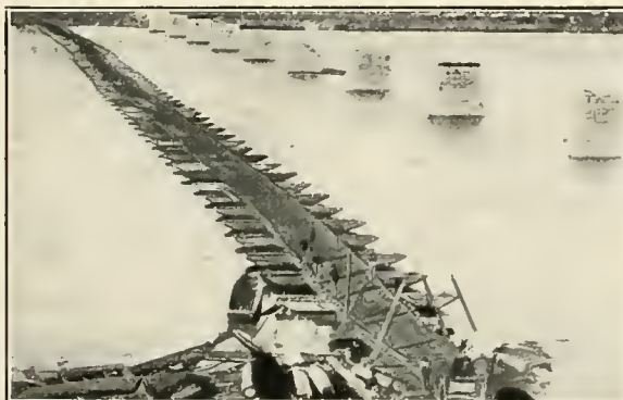
PONTOON-BRIDGE AT DECATUR
