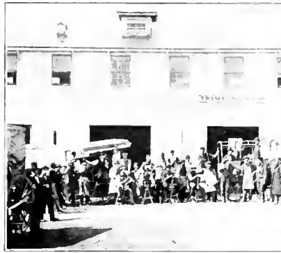
GOVERNMENT TRIMMING SHOP
