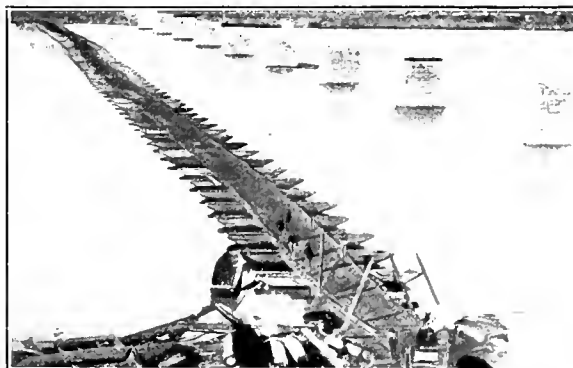
PONTOON-BRIDGE AT DECATUR
