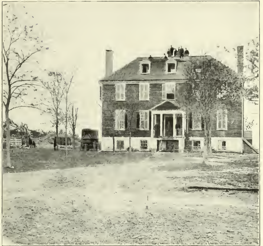
A LOOKOUT ON THE ROOF OF FARENHOLT'S HOUSE, YORKTOWN
