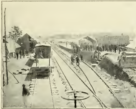
STORES AT STONEMAN'S STATION
