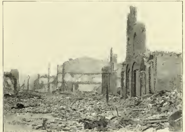
WORK OF THE FLAMES
