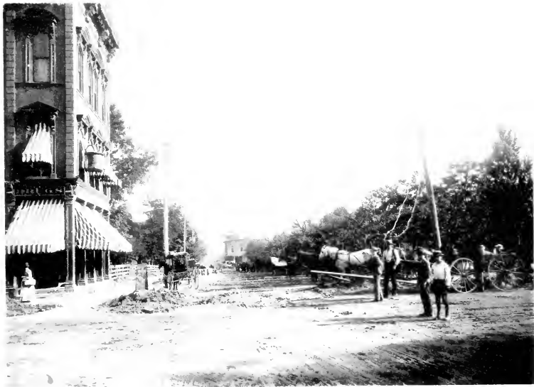
Barr St. Market, Looking North.
