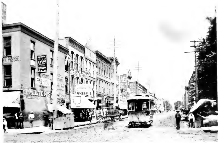
Main St. Looking East from Calhoun Street.
