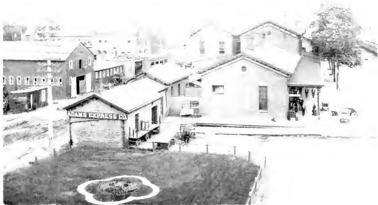
Pennsylvania Rail Road Depot and Streets
