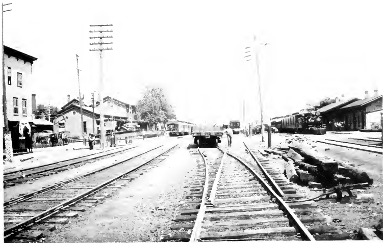
P. Ft. W. & C. and Wabash R. R. Depots
