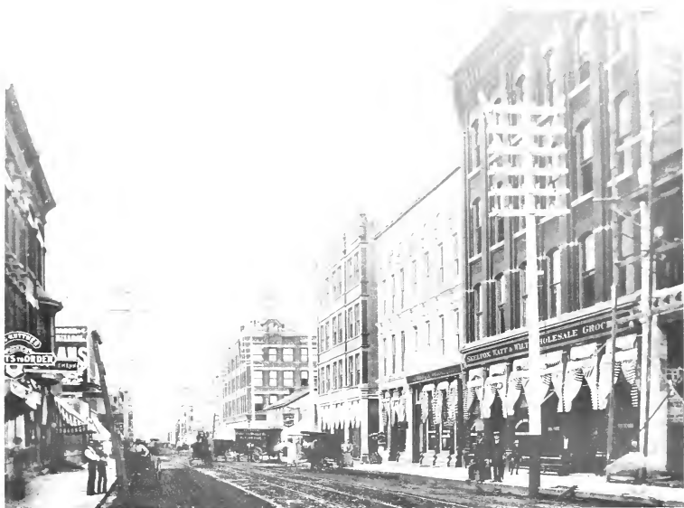
Calhoun St. Looking North from Jefferson St
