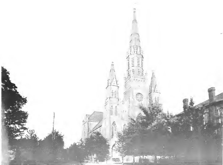
St. Mary's Catholic Church, Cor. Lafayette and Jefferson Sts.
