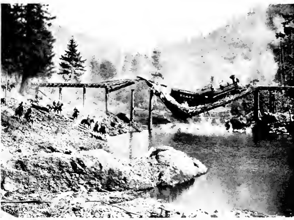
Forty thousand dollars went into the making of this scene for Buster Keaton's comedy, "The General." A locomotive of the Civil War period dashed onto a burning trestle and plunged into the river below. A dozen cameras filmed the scene, while Buster stood nearby without cracking a smile
