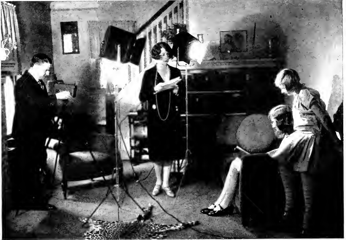
The correct way to shoot an interior. Source of illumination is placed at an approximate angle of 45 degrees about subjects. The camera, a Cine-Kodak, shoots between, while the Kirbylites are directed at their nearest subjects, thus properly lighting scene. The light toned walls help
