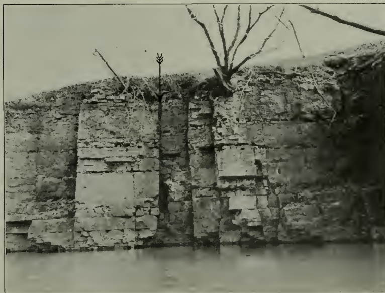
B. Fault in the Wall of Sugar Creek Gorge. The fault fracture cuts the large rectangular opening. The block on the right is a foot above that on the left.
