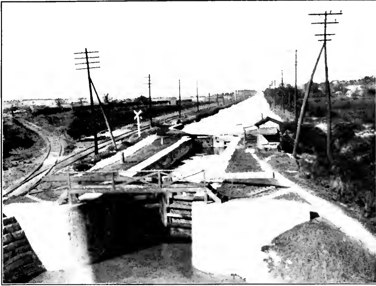
A. Lock on the Illinois-Michigan Canal, above Joliet.
