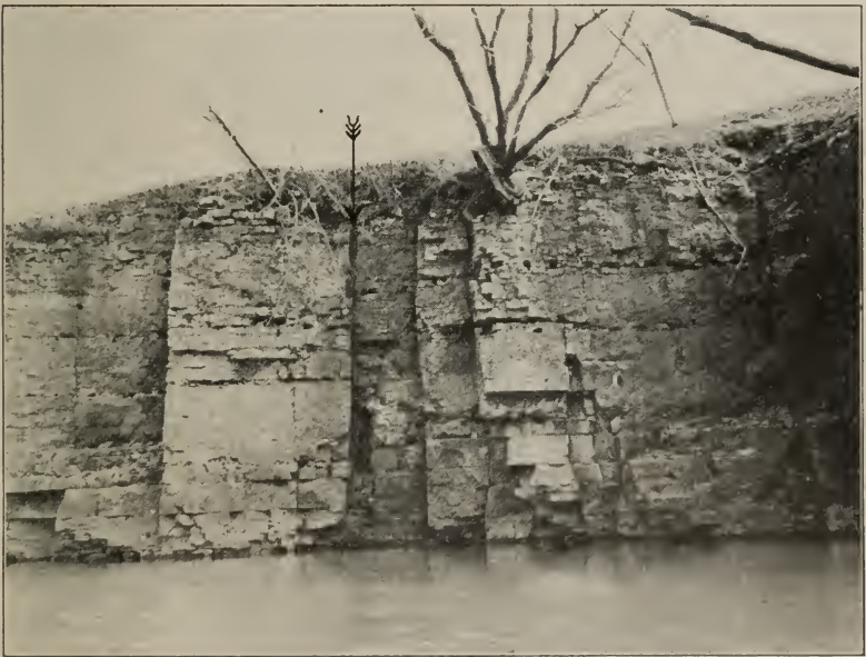
B. Fault in the Wall of Sugar Creek Gorge. The fault fracture cuts the large rectangular opening. The block on the right is a foot above that on the left.
