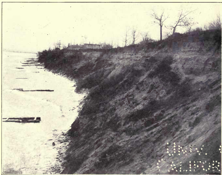
Fig. B. Lake cliff at Racine, Wis., near Racine College. The waves have continued to encroach upon the land in spite of the piers. [Courtesy of C. & N. W. Ry.]
