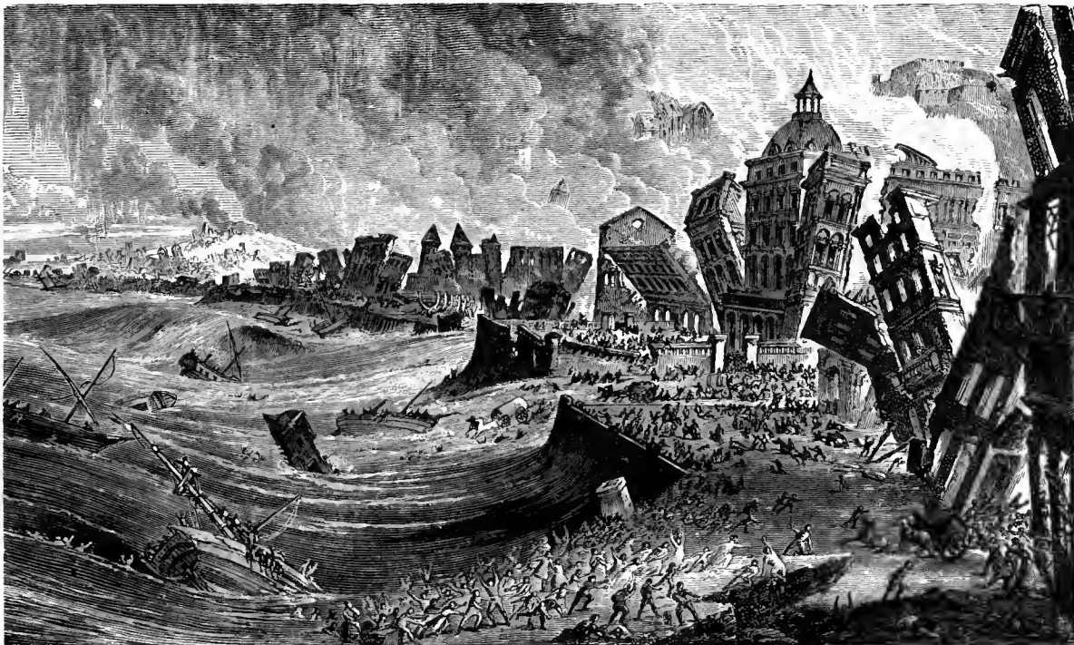
EARTHQUAKE AT LISBON.
