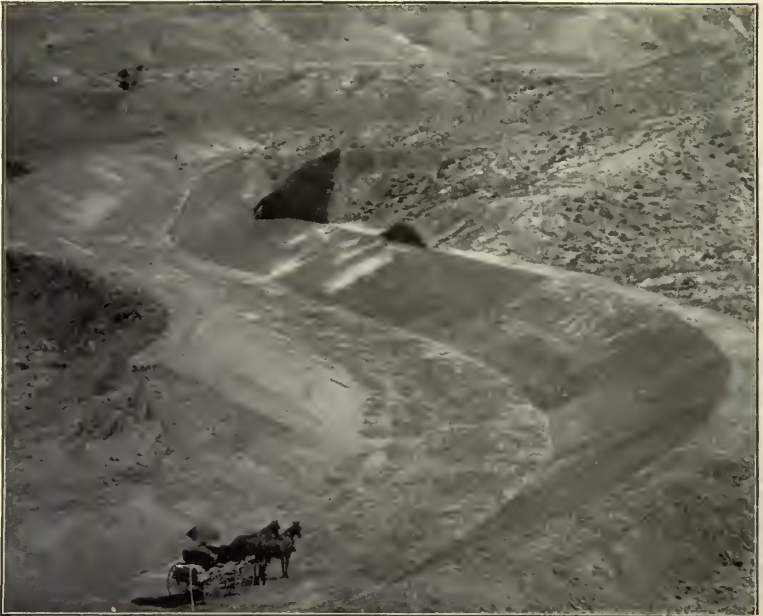
FIG. 199.—An irrigating canal not cemented, before the water is turned in. Salt River Valley, Ariz. (U. S. Geol. Surv.)
