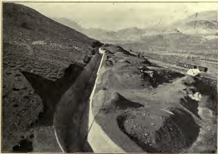
FIG. 198.—A cement-lined canal prepared for irrigation. Truckee-Carson project, Nev. The cement lining prevents free seepage. (U. S. Geol. Surv.)
