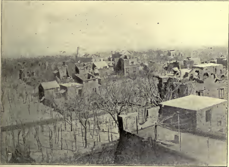
FIG. 371.—The ruins of Ottajano. The roofs have fallen in under the load of ashes.
