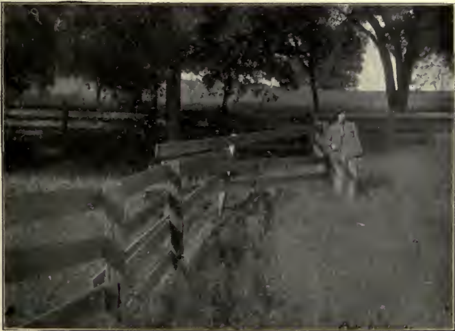
FIG. 456.—A broken (now mended) and offset fence. That in the foreground was formerly in line with the single length directly behind the man.
