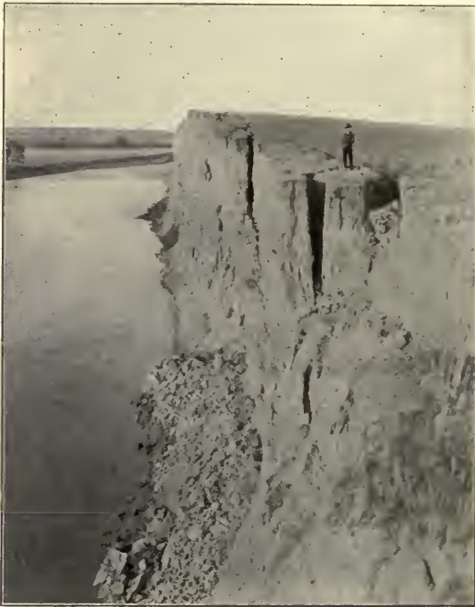
FIG. 98.—Material settling off the face of a cliff under the influence of gravity. The freezing of water in the cracks may be a factor in the separation of the cliff face. (U. S. Geol. Surv.)
