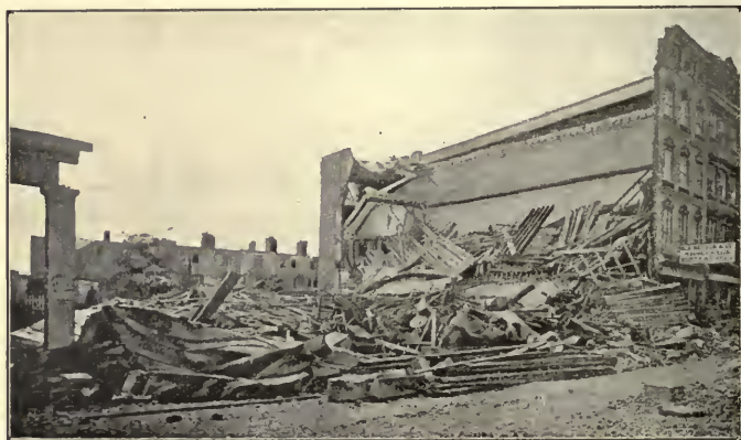
FIG. 446.—Wreck of the Charleston earthquake. (U. S. Geol. Surv.)
