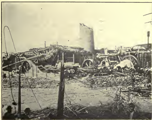
FIG. 658.—Wreckage of the Union Station Power-house at St. Louis, May 27, 1896. (U. S. Weather Bureau.)
