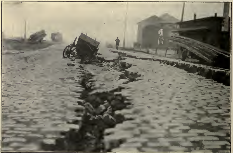
FIG. 454.—A fissure on East Street, San Francisco, near the water front. "Made" ground. (Lindgren, U. S. Geol. Surv.)
