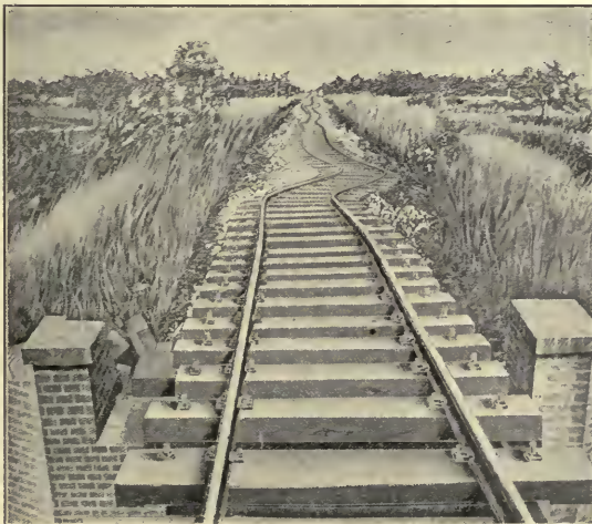
FIG. 441.—The bending of railway track in India, earthquake of 1897. (Oldham.)
