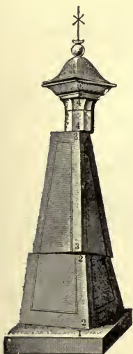
FIG. 435.—Monument disturbed by earthquake. (Falb.)
