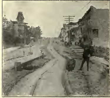
FIG. 460 B.—A street railway on loose ground. Union Street, near Pierce Street. (Photo. by Moran.)
