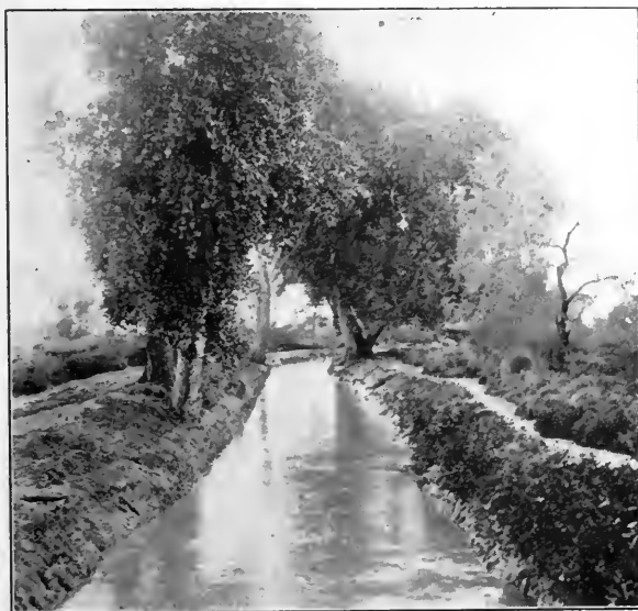
FIG. 201.—An irrigating canal filled with water. Salt River Valley, Ariz. (U. S. Geol. Surv.)
