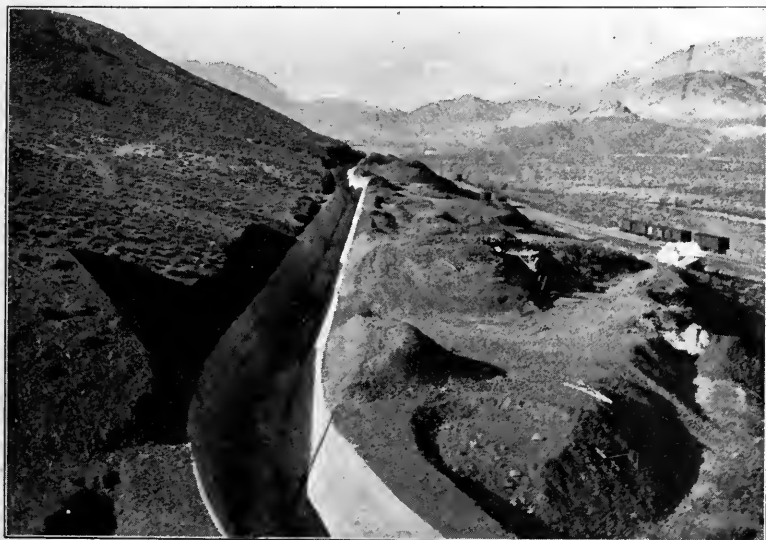
FIG. 198.—A cement-lined canal prepared for irrigation. Truckee-Carson project, Nev. The cement lining prevents free seepage. (U. S. Geol. Surv.)
