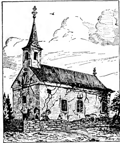
FIG. 436.—A chapel in Kasina injured in an earthquake of November 9, 1880. (Wähner.)
