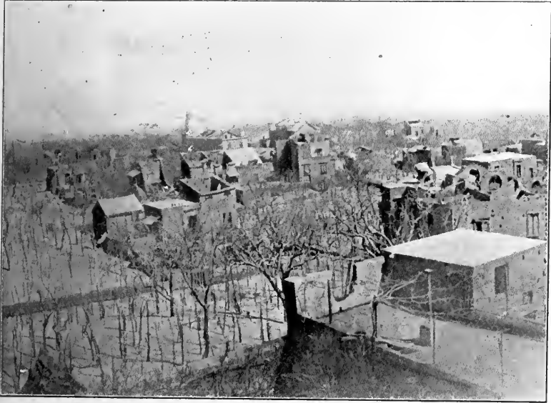
FIG. 371.—The ruins of Ottajano. The roofs have fallen in under the load of ashes.
