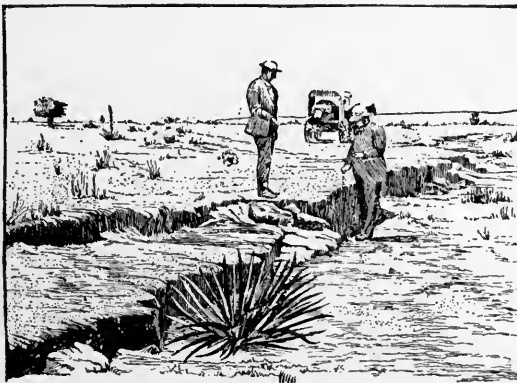
FIG. 467.—Fissure produced by earthquake. Arizona.
