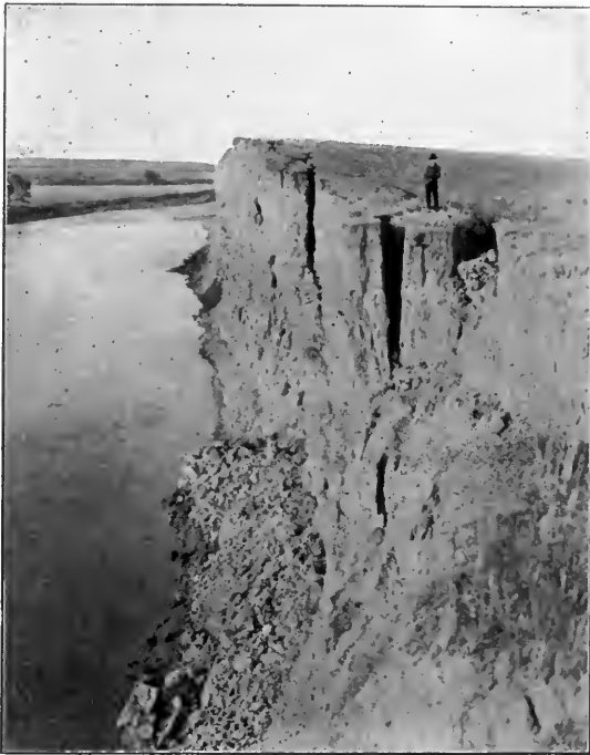
FIG. 98.—Material settling off the face of a cliff under the influence of gravity. The freezing of water in the cracks may be a factor in the separation of the cliff face. (U. S. Geol. Surv.)
