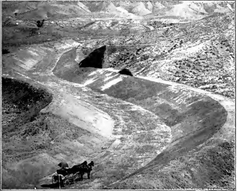
FIG. 199.—An irrigating canal not cemented, before the water is turned in. Salt River Valley, Ariz. (U. S. Geol. Surv.)
