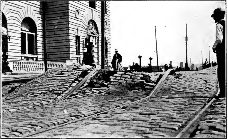
FIG. 453.—Deformed railway, Seventh and Mission Streets, San Francisco. (Lindgren, U. S. Geol. Surv.)
