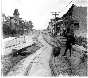
FIG. 460 B.—A street railway on loose ground. Union Street, near Pierce Street. (Photo. by Moran.)
