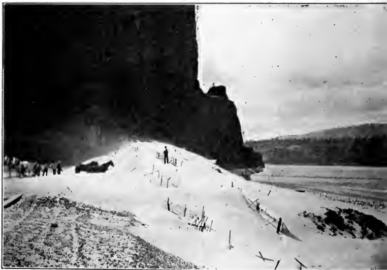
FIG. 61.—Sand drifted over railway. Rowena, Wash. (Dept. of Agr.)
