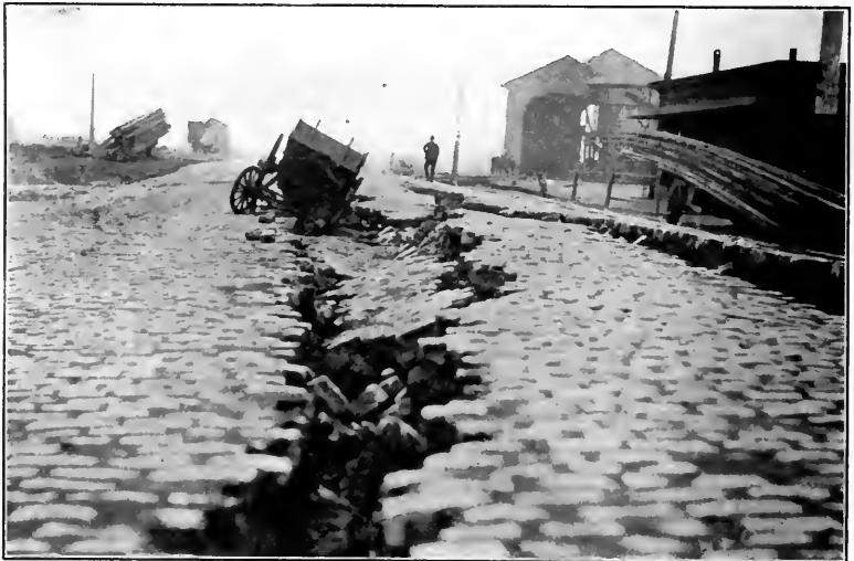
FIG. 454.—A fissure on East Street, San Francisco, near the water front. "Made" ground. (Lindgren, U. S. Geol. Surv.)
