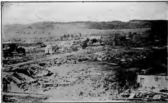
FIG. 657.—General view of the wreckage caused by the tornado at Rochester, Minnesota, August 21, 1883.
