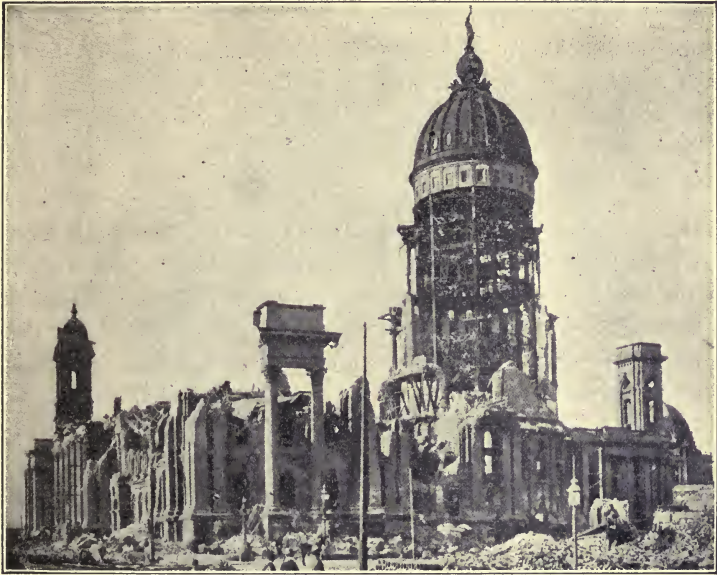
FIG. 230.—RUIN OF THE $7,000,000 CITY HALL BY THE SAN FRANCISCO EARTHQUAKE AND FIRE
