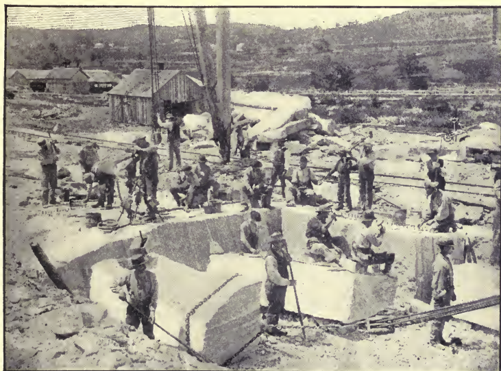
FIG. III.—A GRANITE QUARRY
