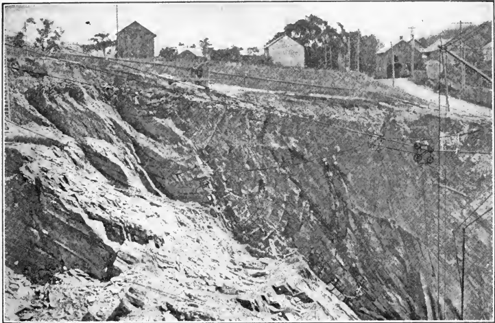
FIG. 114.—A SLATE QUARRY Slatington, Pa.
