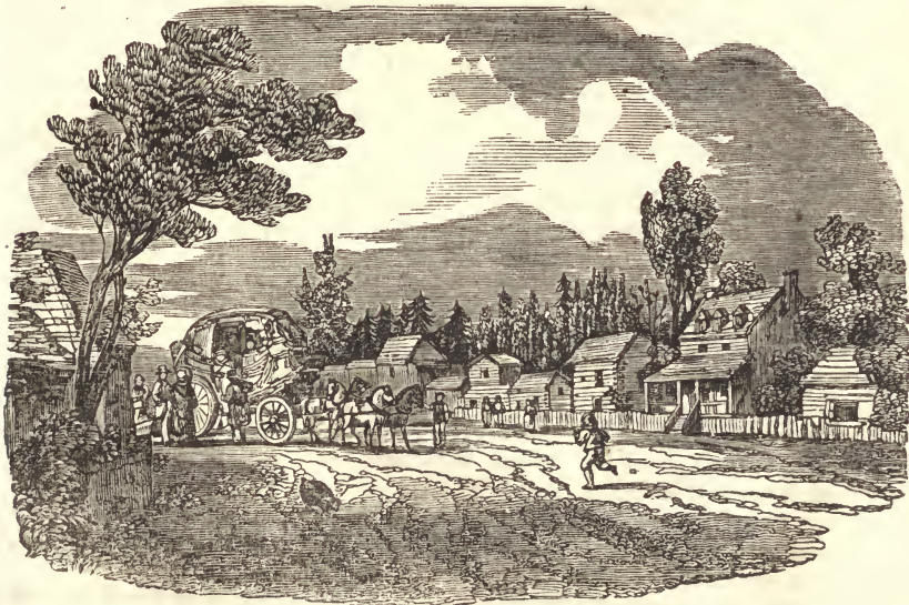
FIG. 121.—Village of Log-Huts.
