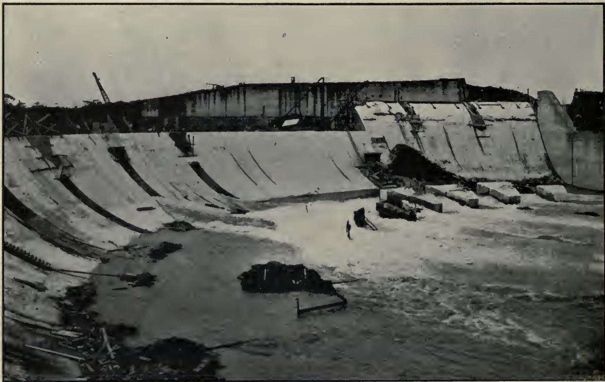
Gatun Spillway Looking Southwest, Showing Downstream Face of Ogee Dam, as it Appeared June 6, 1912.
