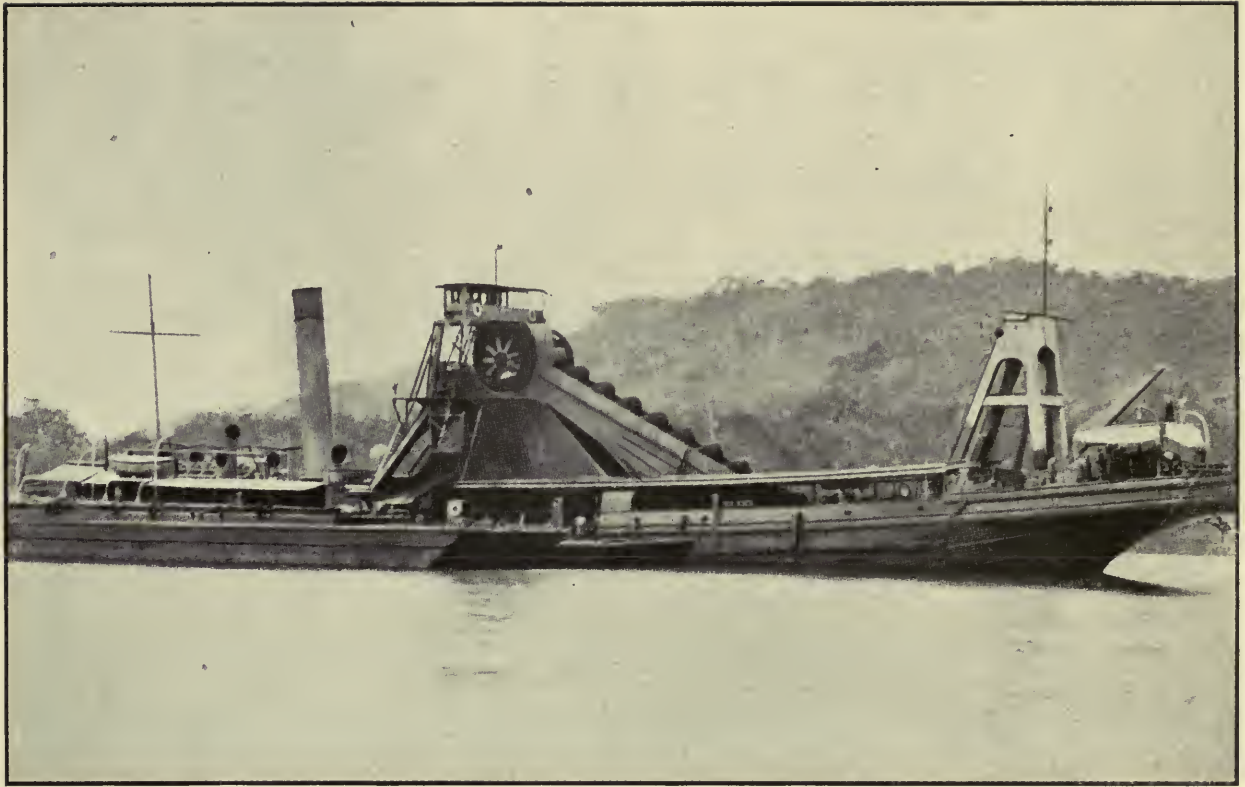
Dredge "Corozal" in Channel Near Station 2210 of the Canal Operations. Photographed in June, 1912.
