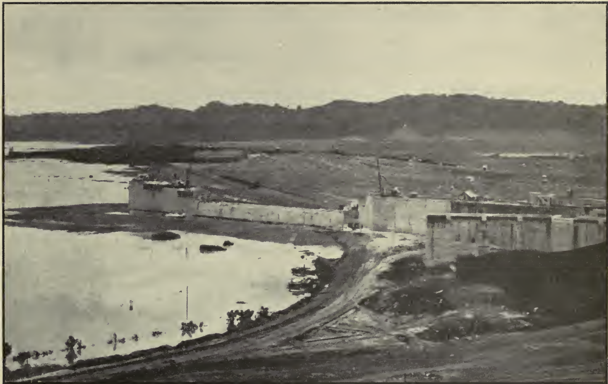
Gatun Locks and Dam, Looking West from Water Tower, Showing South Center Approach Wall and Forebay of Gatun Locks, with Dam and Spillway in the Distance. Photographed June, 1912.
