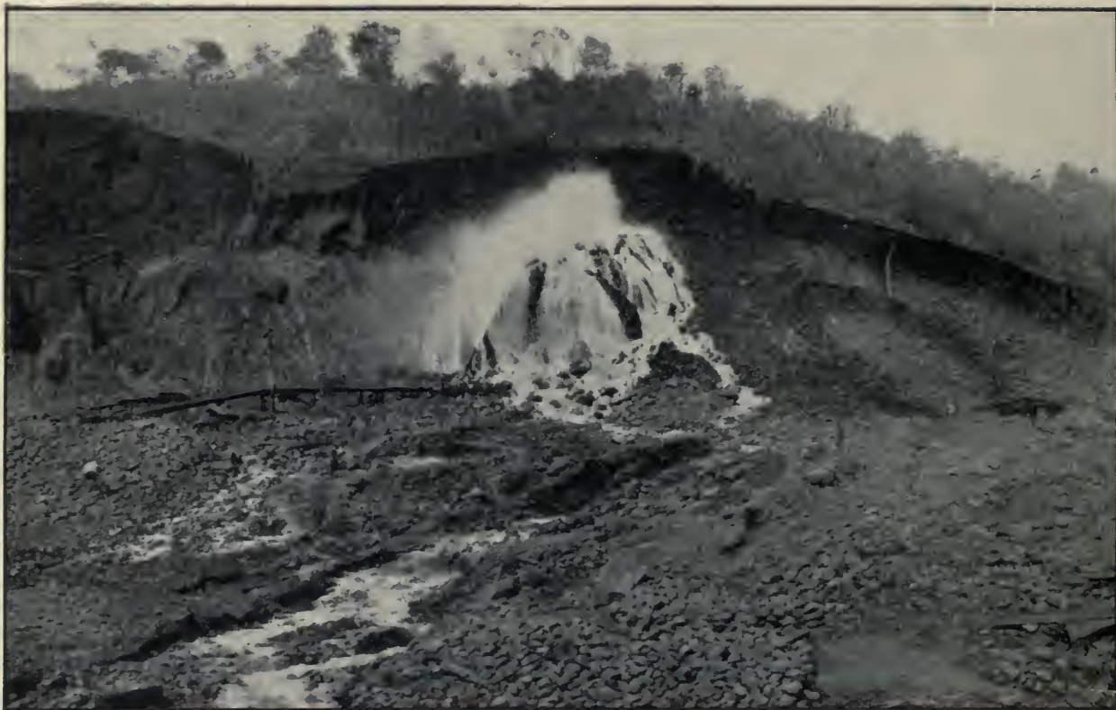
Stripping Cocoli Hill Adjacent to Canal Prism. Photographed March 21, 1912, and Showing the Method of Hydraulic Excavation.
