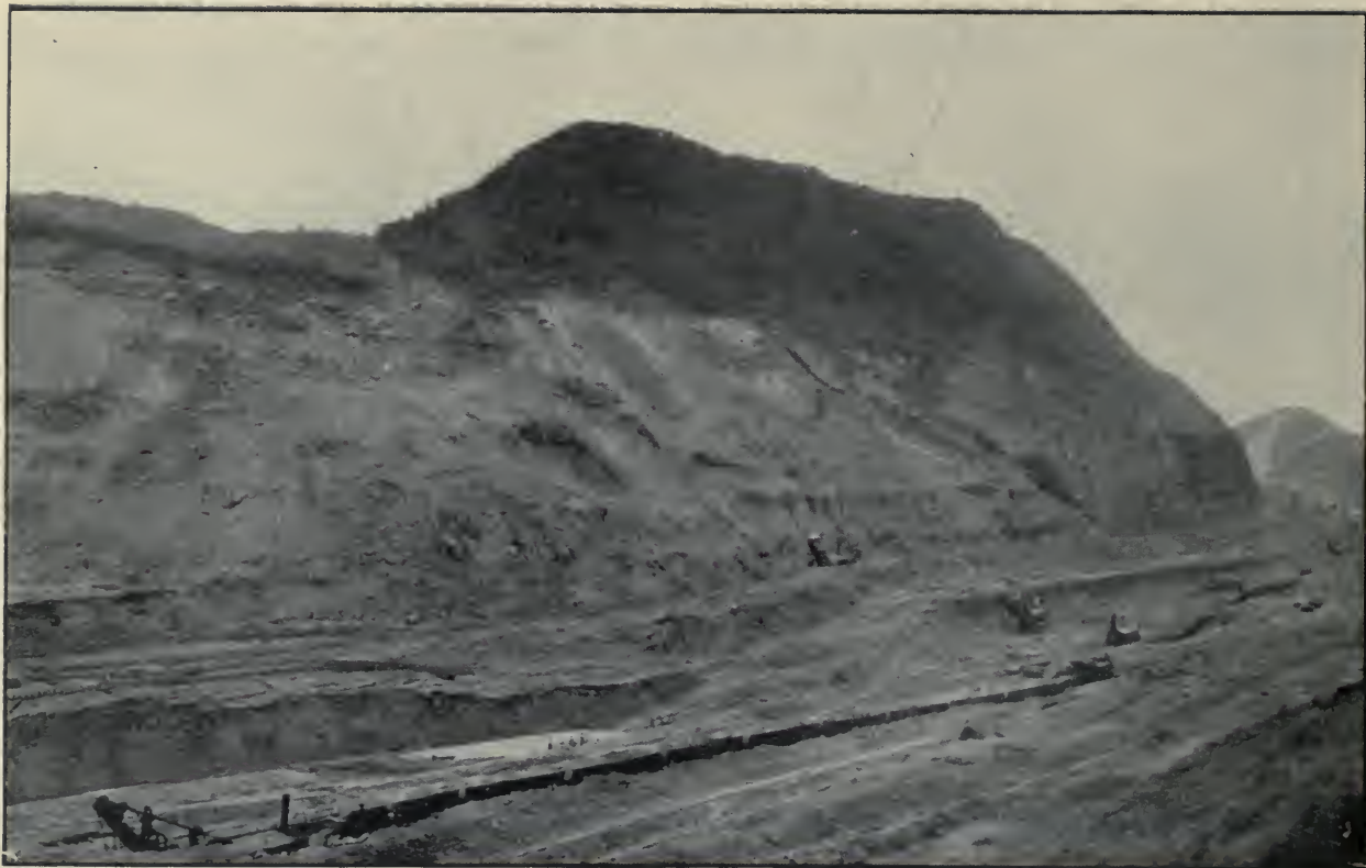
Culebra Cut, Culebra. Break in East Bank of Canal. Amount of Material Involved, 320,000 Cubic Yards. The Train Shown in Foreground Is About 35 Feet Above the Bottom, or at Elevation +75. Photographed February 11, 1912.
