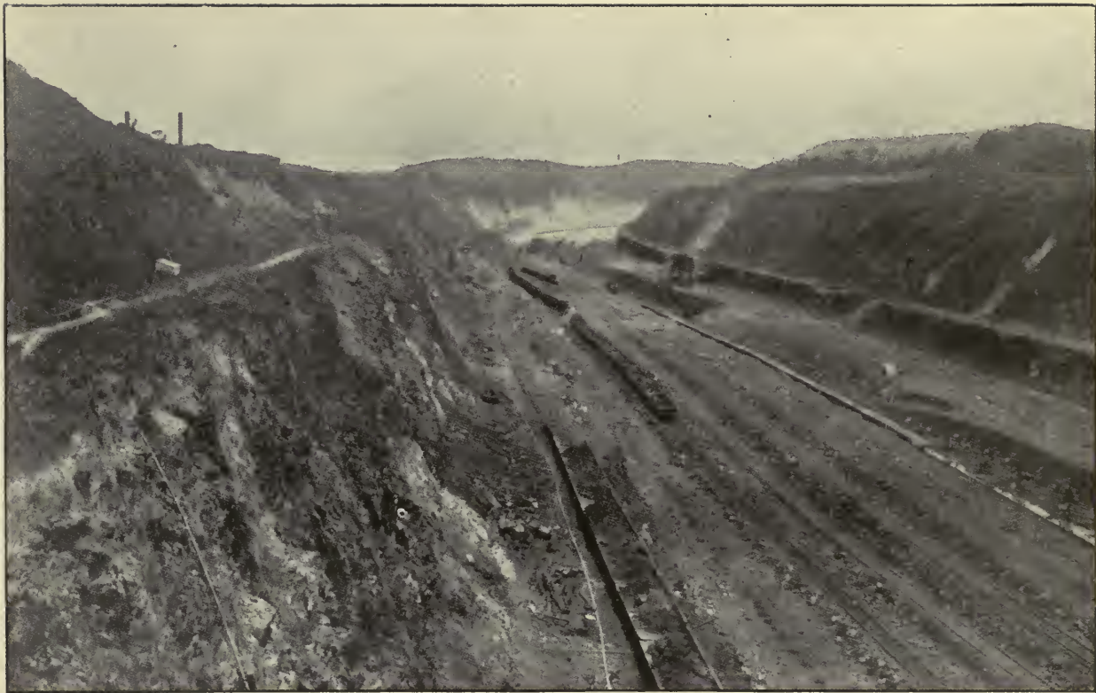
Culebra Cut, Looking North from Empire Suspension Bridge. The Nearest Shovel Shown, in the Lowest Cut, Is Working About 12 Feet Above the Bottom, or at Elevation +52 . The Photograph Was Taken in May, 1912.
