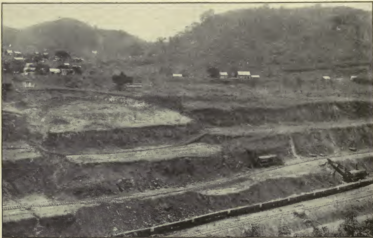
Slide in East Bank of Canal Near Cucaracha, June, 1912. This Illustrates One of the Difficulties with Which the Engineers and Construction Department Have Had to Contend.
