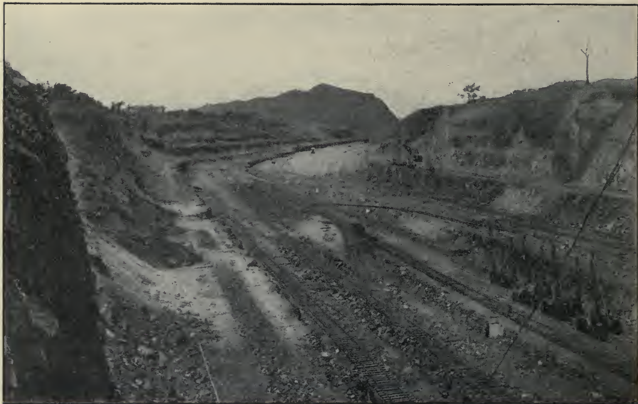
Culebra Cut, Looking South from Empire Suspension Bridge. The Group of Well Drills in the Middle of the Canal Is About 27 Feet Above the Bottom, or at Elevation +67, Photographed May, 1912.
