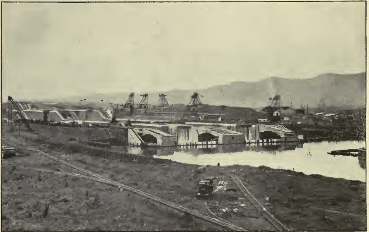
Gatun Locks. General View Looking Southwest, Showing North End of the Locks, with Temporary Cofferdam in Place. Photographed July 2, 1912.
