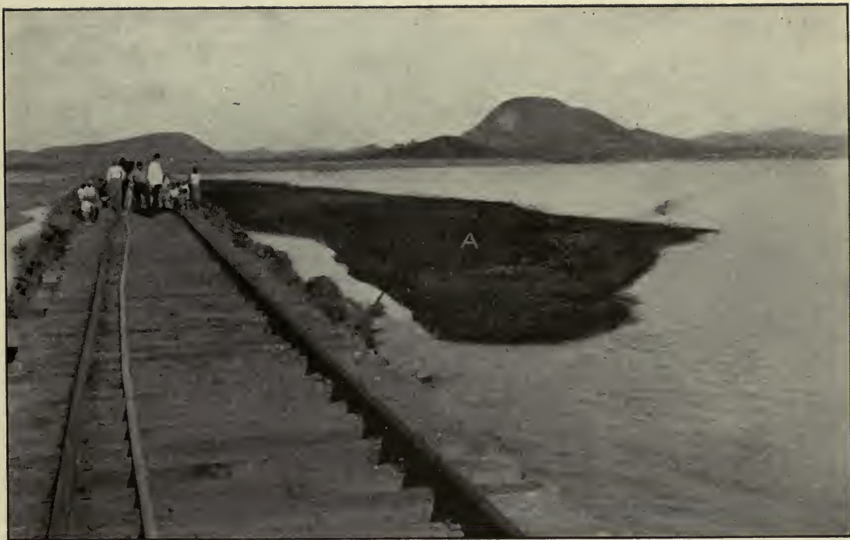
South End of Naos Island Dump, 4,000 Feet from Island. Center at "A" is 75 Feet from Track and 25 Feet Above the Original Bottom. Elevation of Trestle, +14. Photographed December, 1911.
