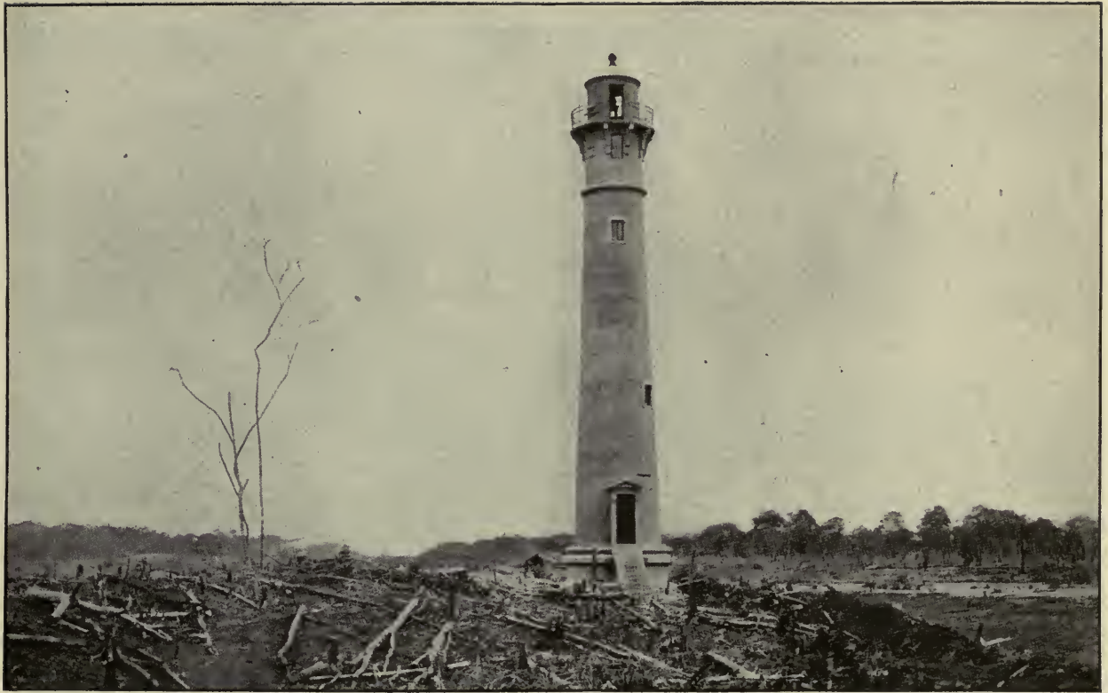
Front Tower, Range 5-6, Atlantic Division. These Range Lights Form an Important Feature of the Navigation Facilities of the Canal System.
