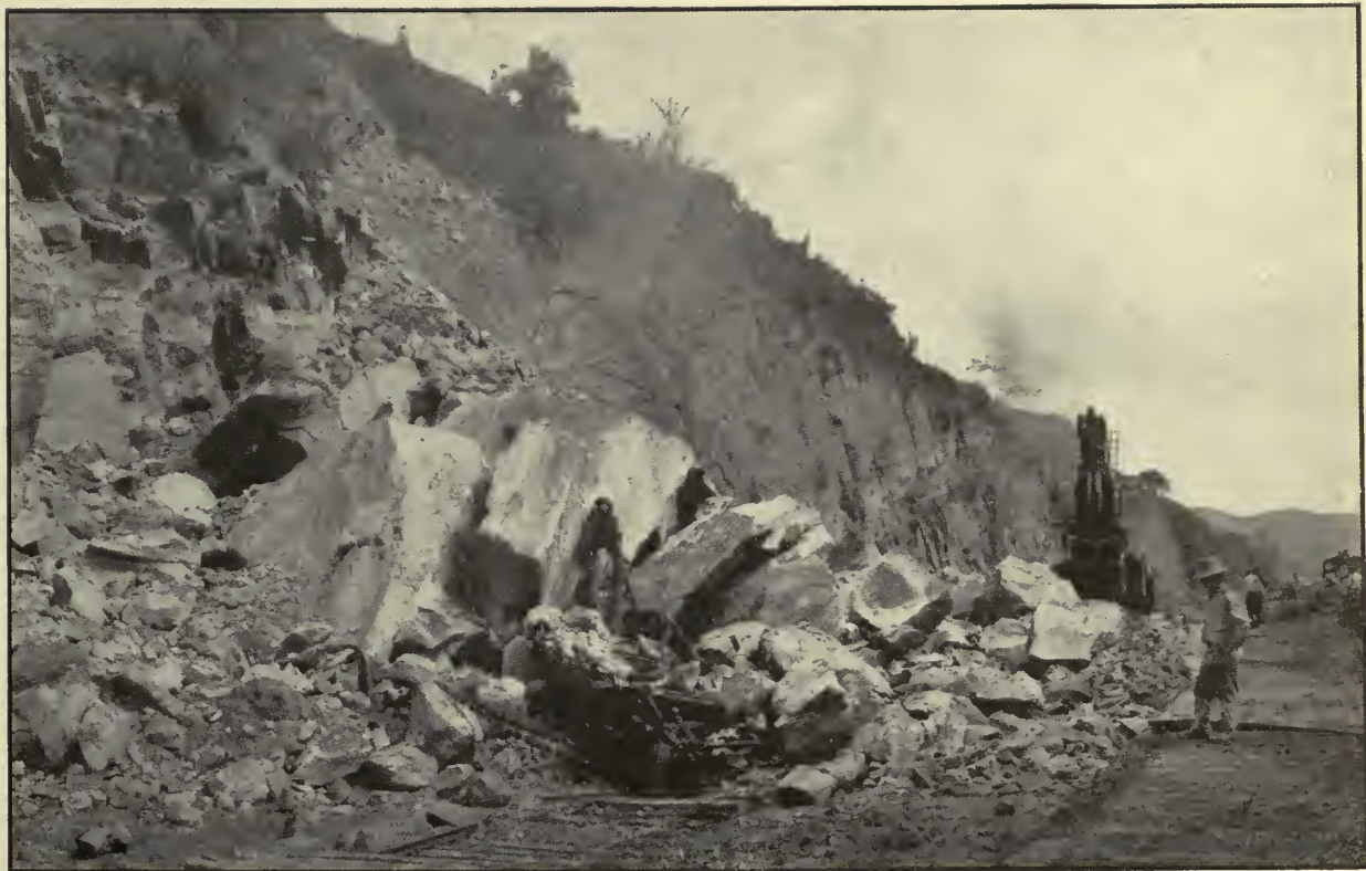
Steam Shovel 218 Buried Under Fall of Rock, West Side of Canal, Near Las Cascadas. This Shovel Was Working on the Bottom of the Canal When Destroyed, May 31, 1912.
