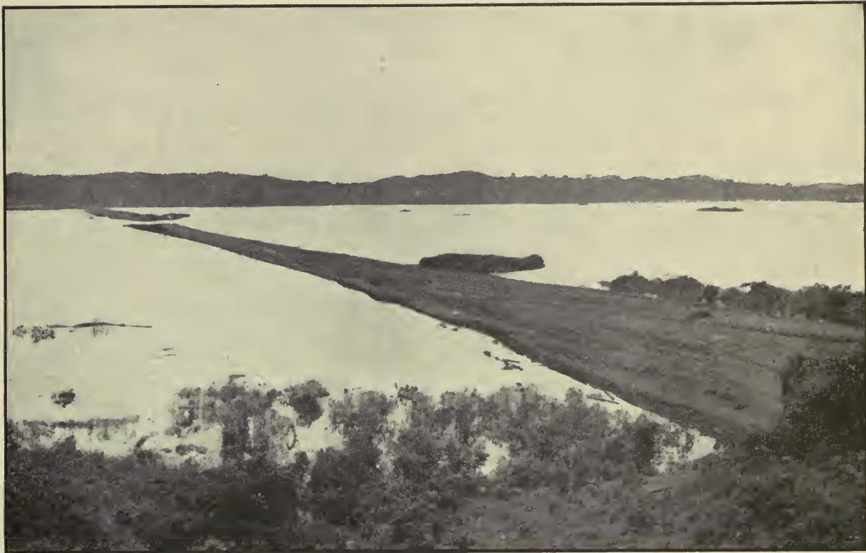
Embankment of Old Panama Railroad Excavated Down to +35 in April and May, 1912.
