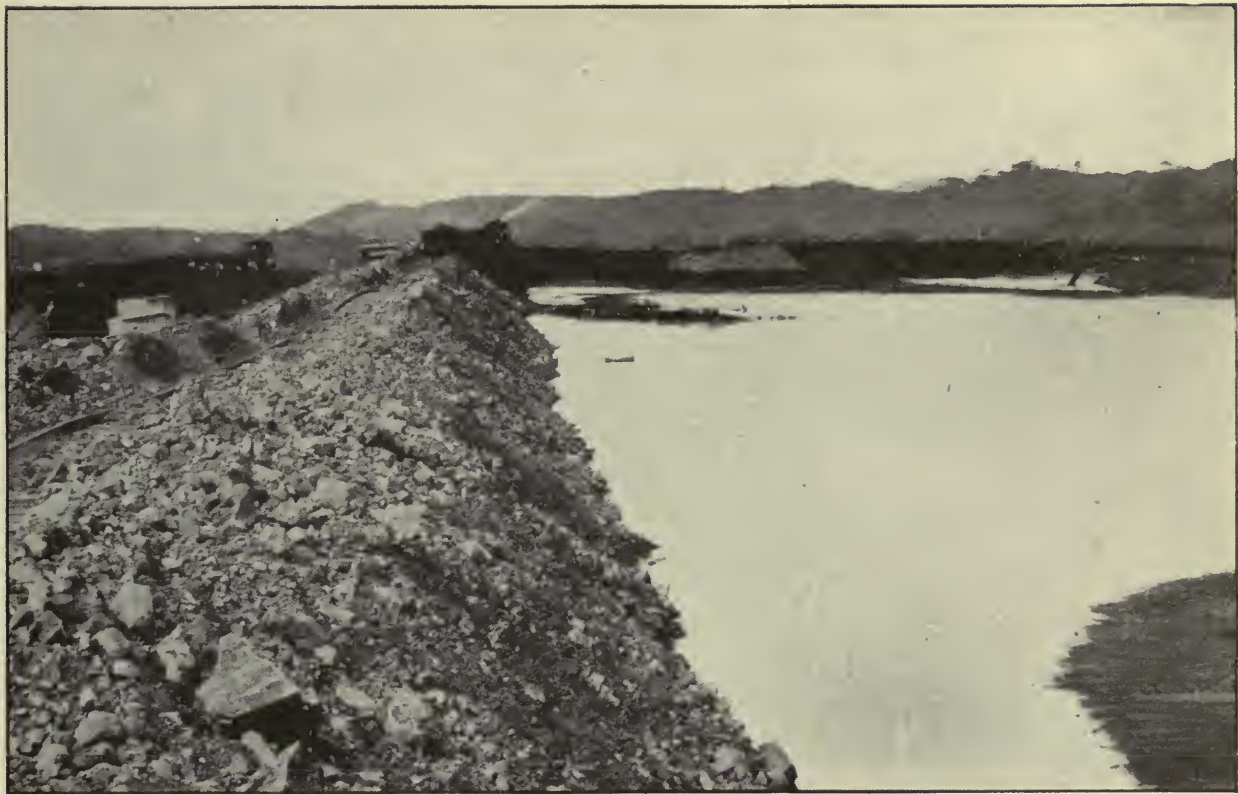
Gatun Dam, West Section of Dam Looking West, Showing Progress of Hydraulic Fill, June 12, 1912. This Great Dam Is Nearly 1\frac{1}{2} Miles Long and About \frac{1}{2} Mile Wide at Its Base.
