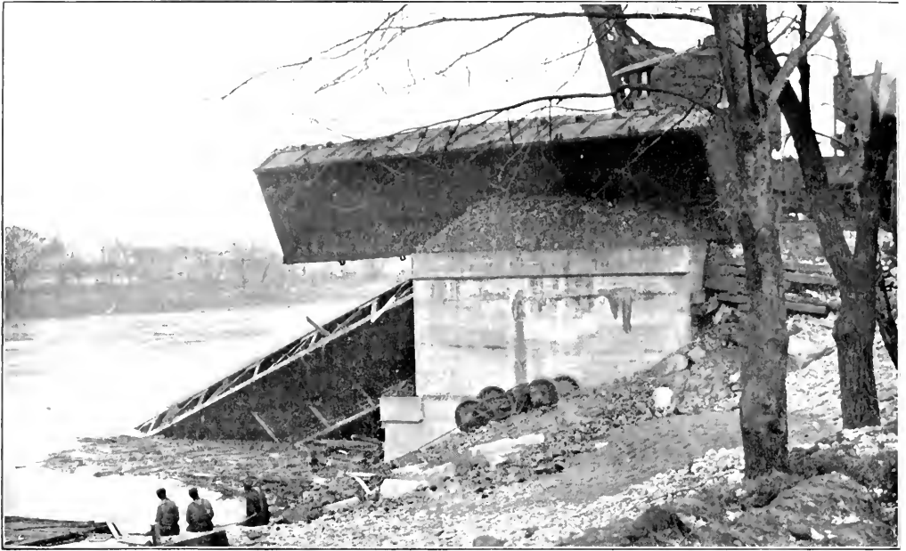
The Railroad Bridge over the Miami
