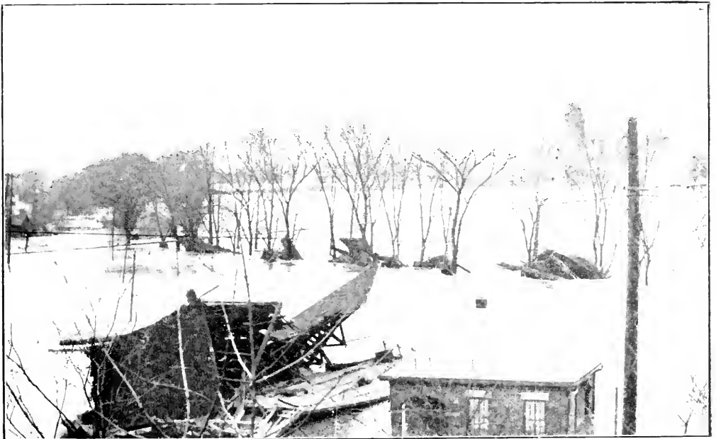
Another View of the Lehman Street Levee.
