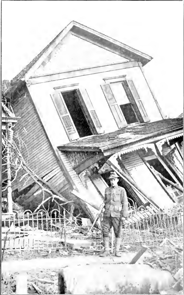
Wrecked House in North Dayton.
