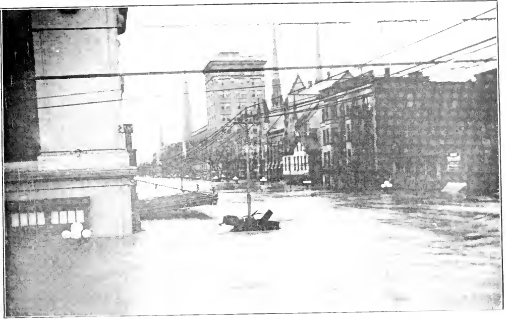
Flood scene looking from Fifth Street north on Ludlow.
