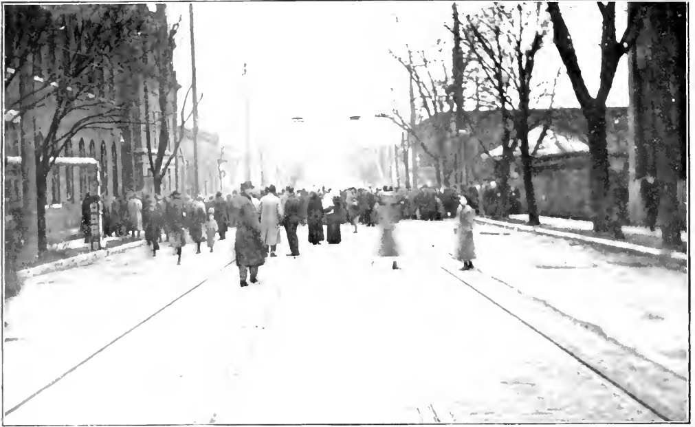
The Western Edge of the Flood on West Third Street Extended to the Malleable Iron Works beyond Conover Street.
