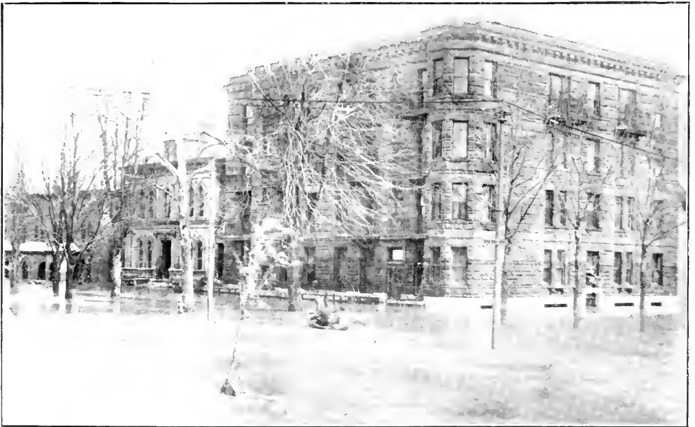
Receding water at the corner of Third Street and Robert Boulevard. Note the high water mark on the building.
