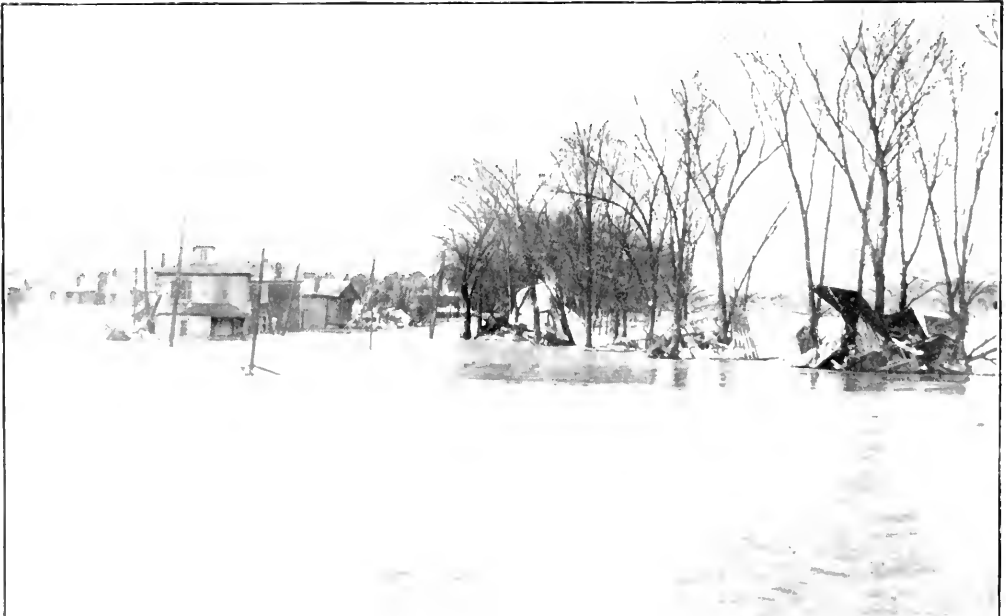
Locking East in Lehman Street and along Riverdale Levee.
