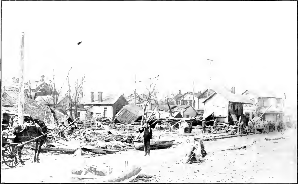
Some of the Destruction on Burns Avenue.
