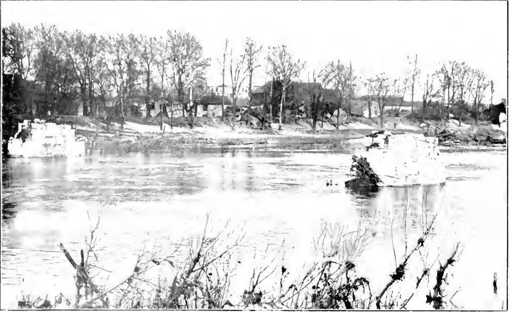
The remains of the West Fifth Street Bridge over the Miami.
