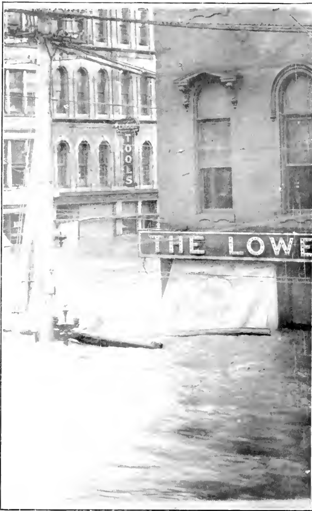
Flood Tide at Third and Jefferson.
