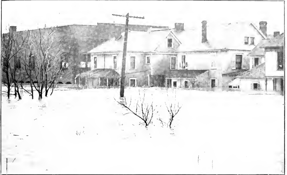
Rear of Grimes Street at Edgewater.
