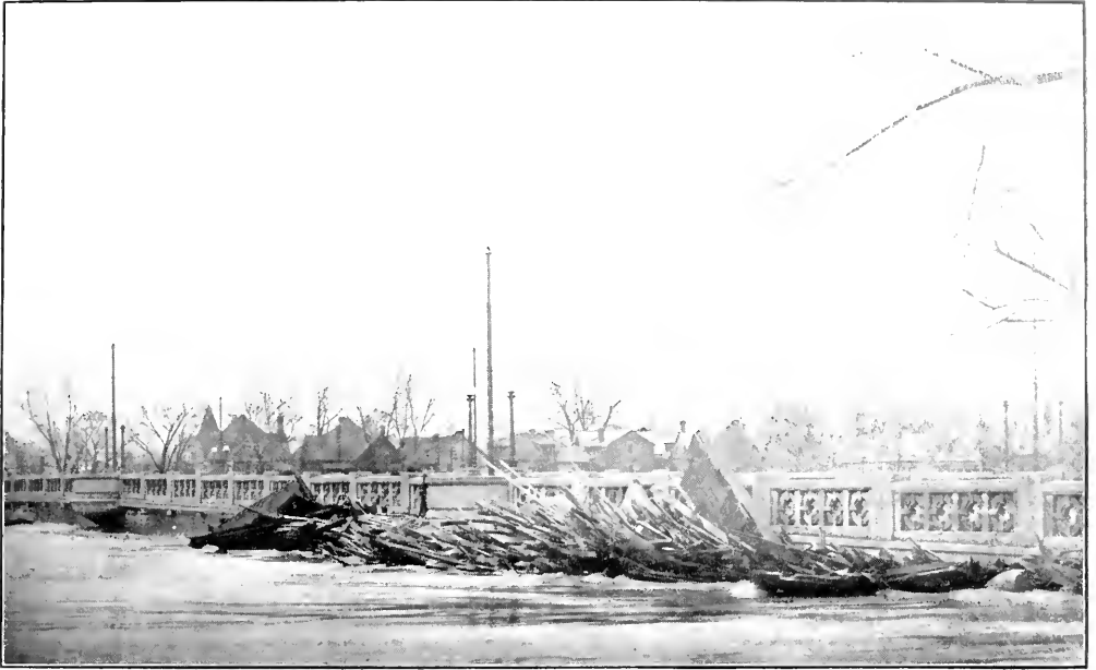
The Up-stream, or East Side of Dayton View Bridge.
