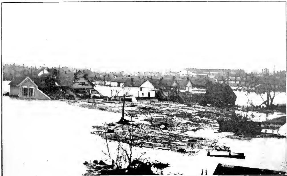
Another Scene of Destruction in North Dayton.
