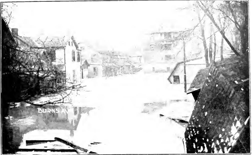
Burns Avenue in Southeast Dayton.
