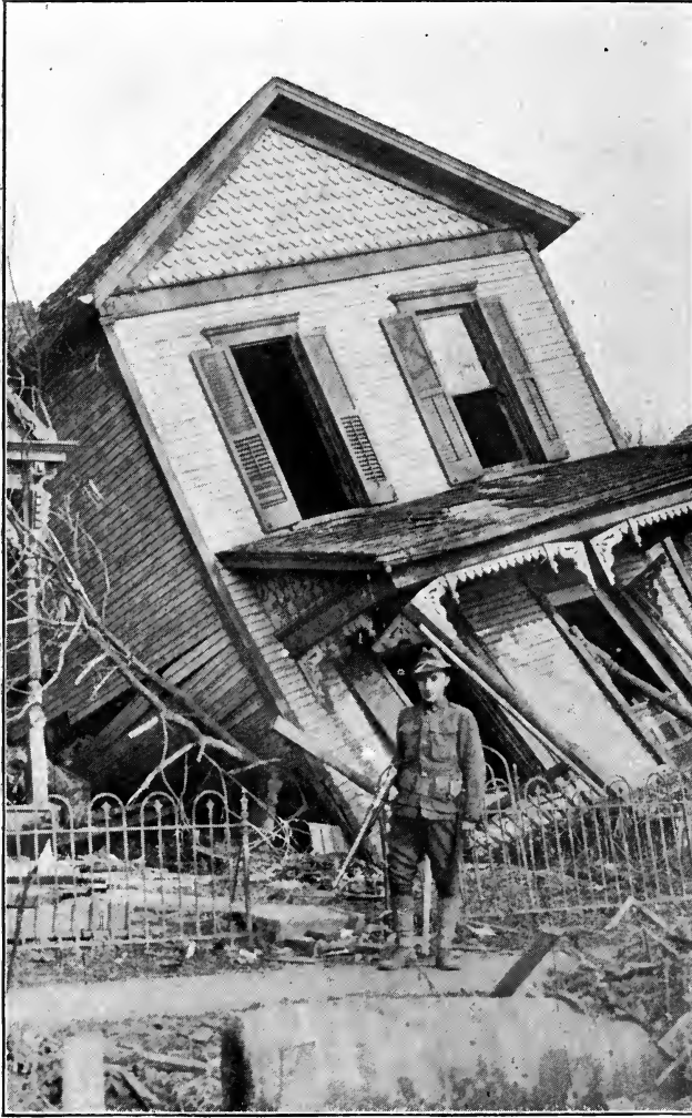
Wrecked House in North Dayton.
