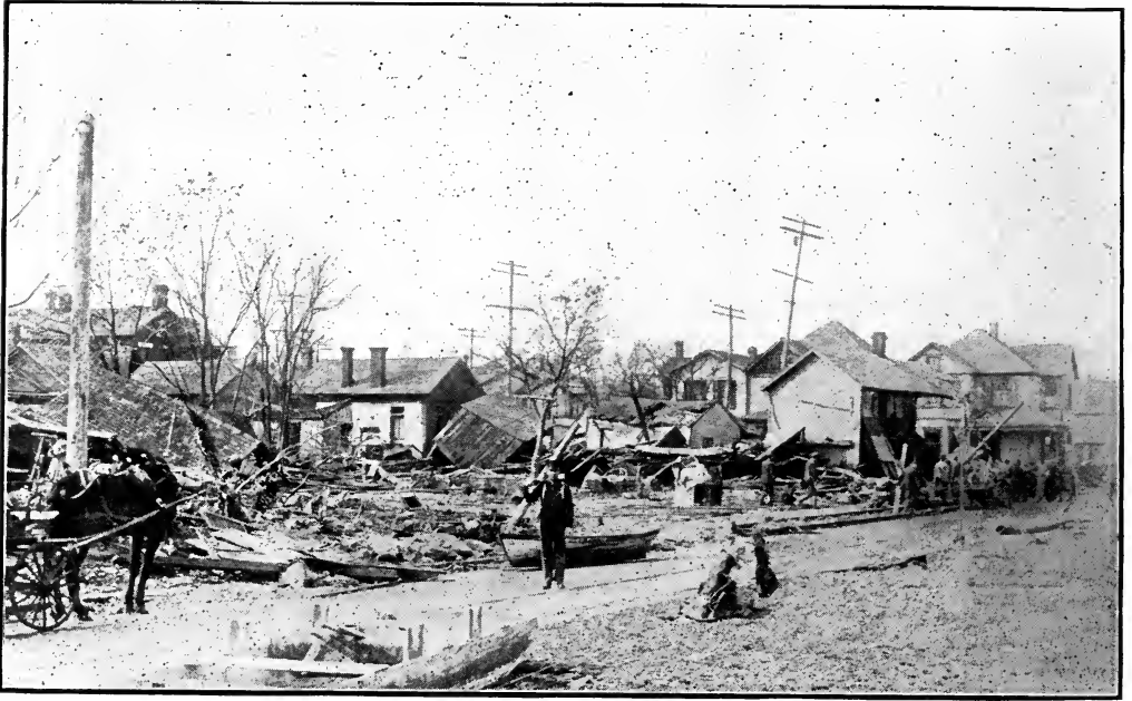
Some of the Destruction on Burns Avenue.
