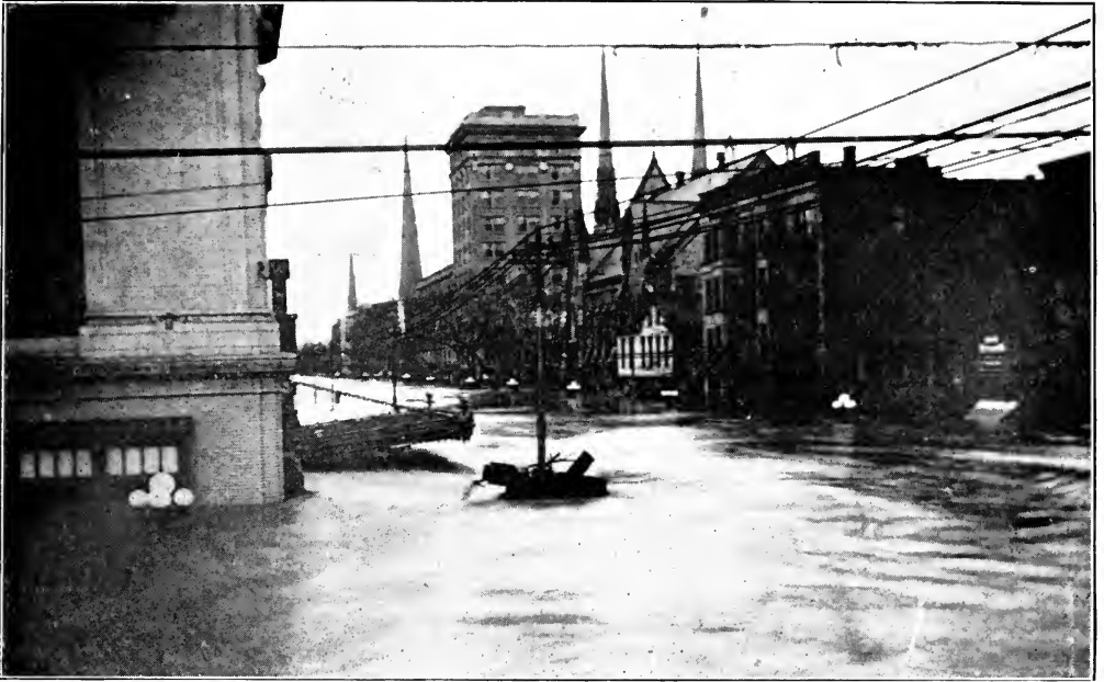
Flood scene looking from Fifth Street north on Ludlow.
