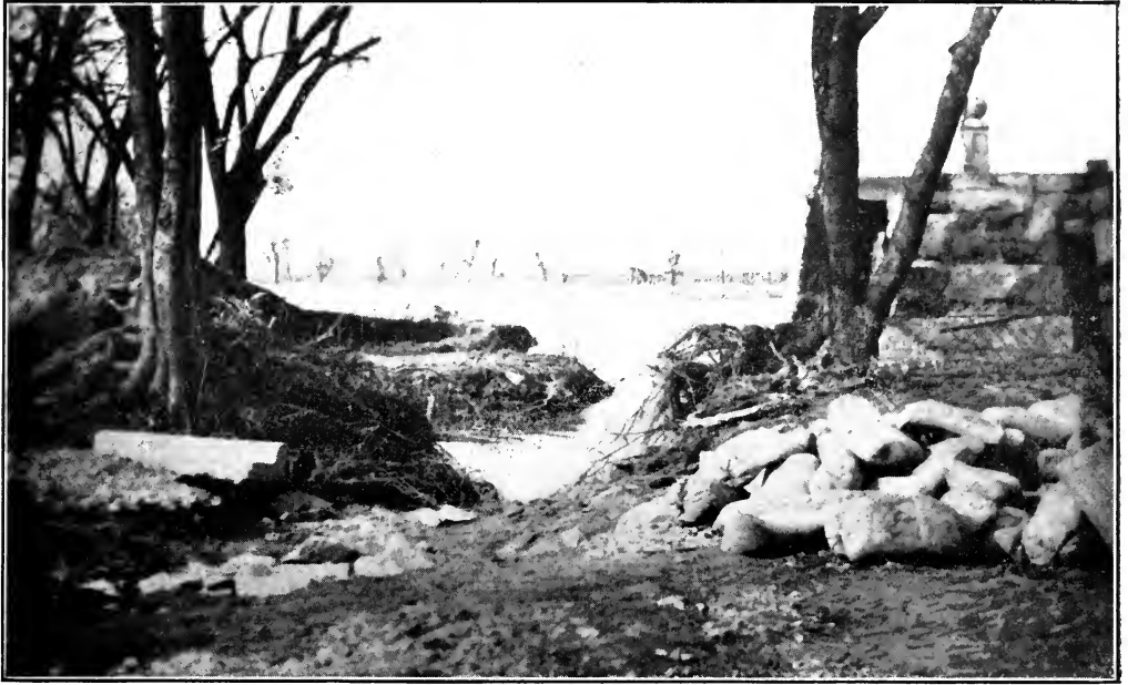
Levee at the Riverdale end of the Steele Dam.
