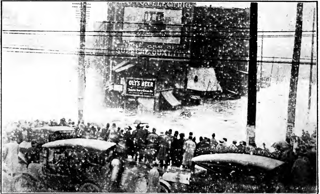
Looking north up the Miami and Erie Canal.
