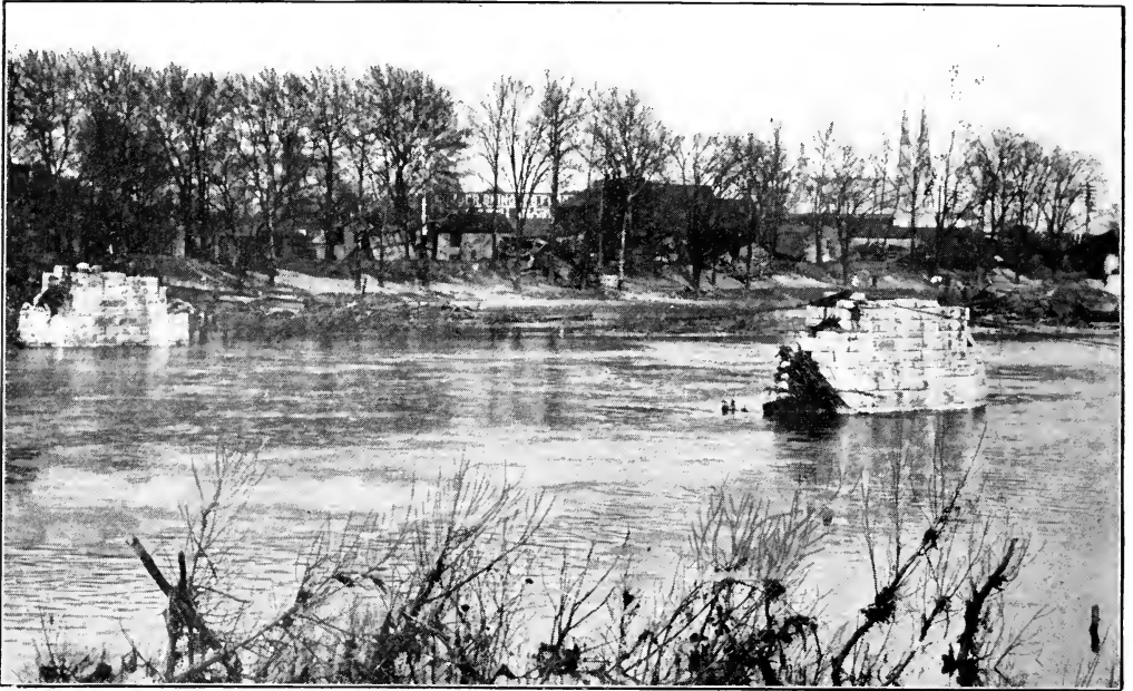
The remains of the West Fifth Street Bridge over the Miami. Our steel concrete bridges held like adamant and one of this sort will replace this old steel and masonry type.
