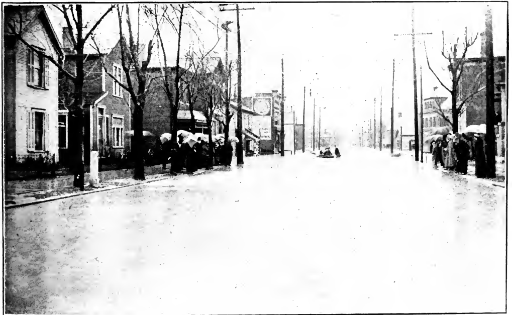
Showing Rescue Work in South Brown Street.
