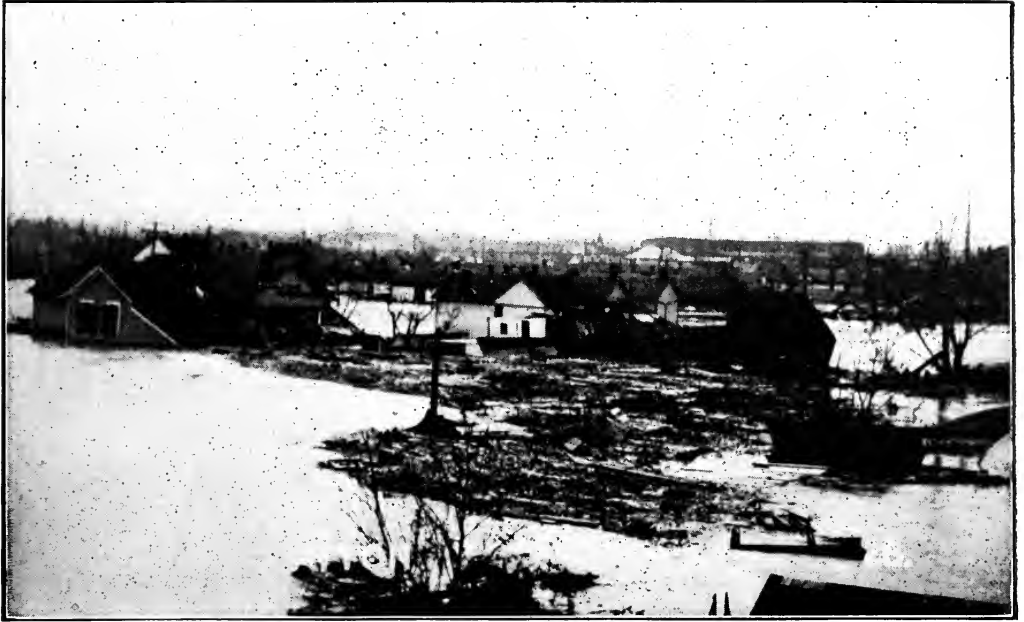
Another Scene of Destruction in North Dayton.
