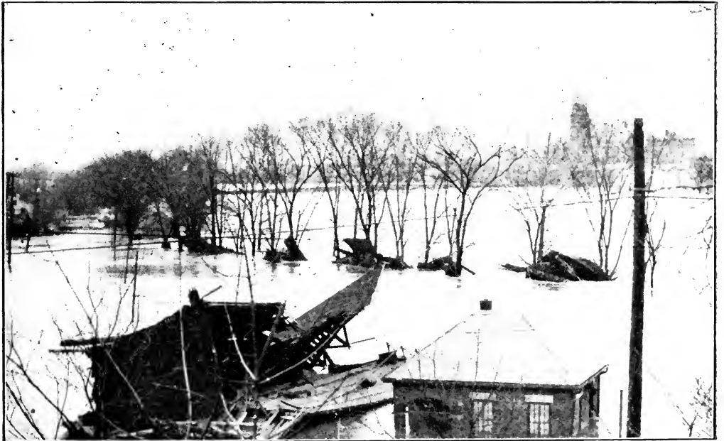
Another View of the Lehman Street Levee.
