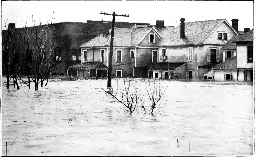
Rear of Grimes Street at Edgewater.
