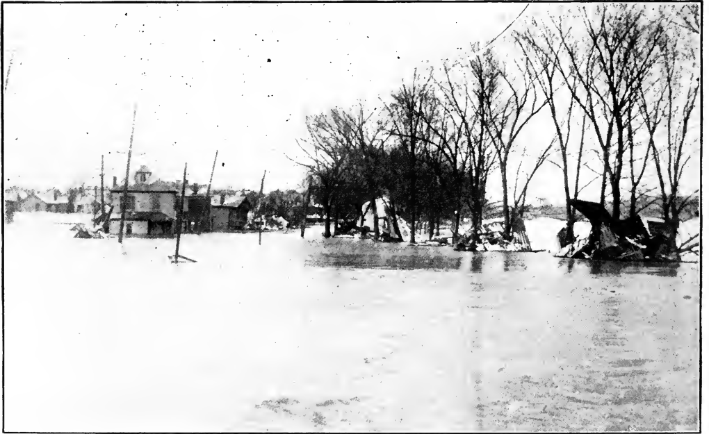
Looking East in Lehman Street and along Riverdale Levee.
