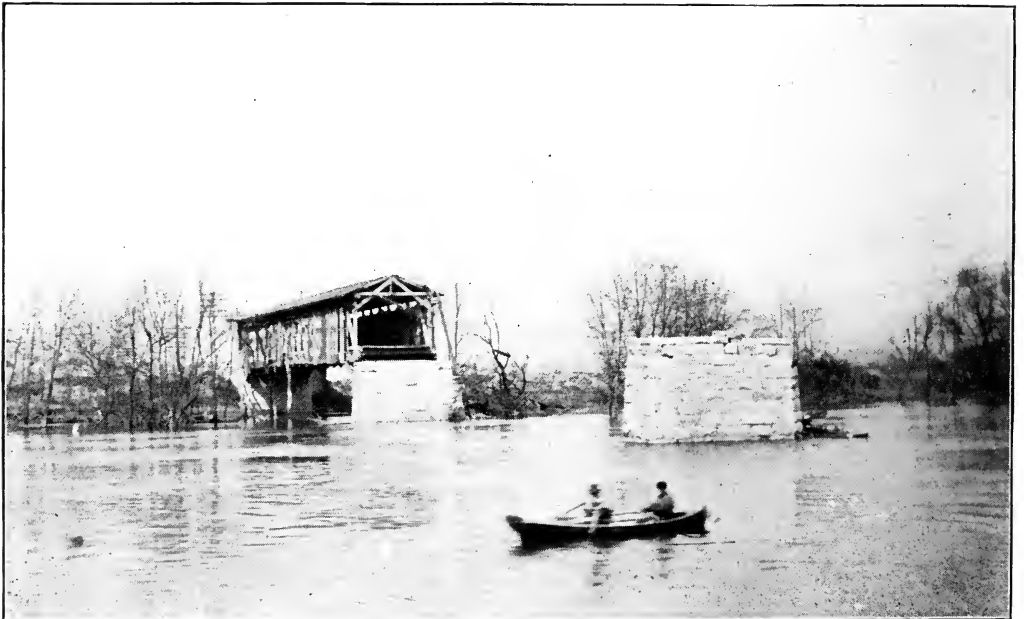
Miller's Bridge, South of Dayton. No chance for such a bridge to outlive the flood.
