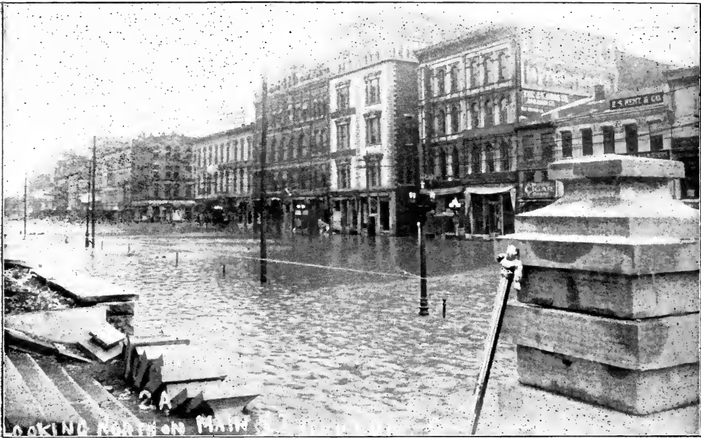
Receding Water in North Main Street.
