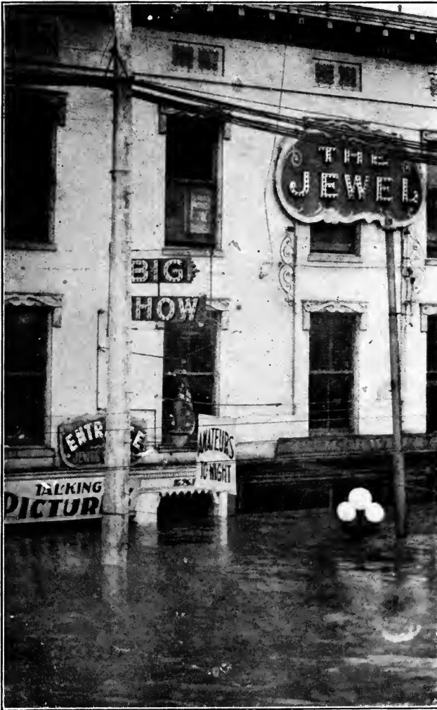
High water in South Jefferson Street.
