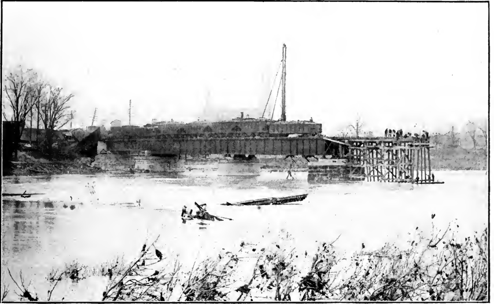
Repairing the Railroad Bridge.
