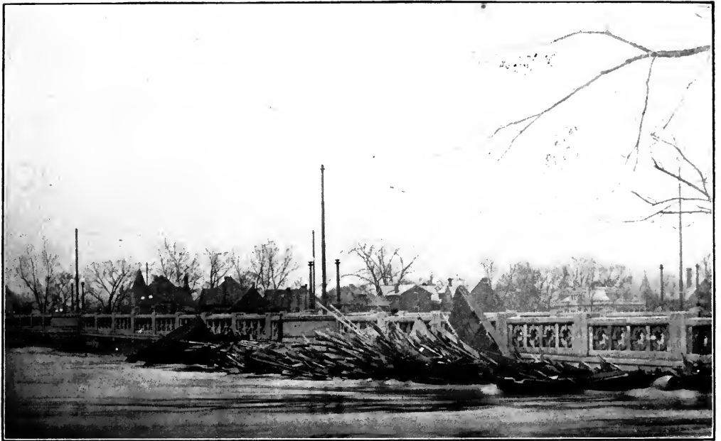
The Up-stream, or East Side of Dayton View Bridge. Showing the flood high above the apertures of the bridge and the latter clogged with wrecked houses.
