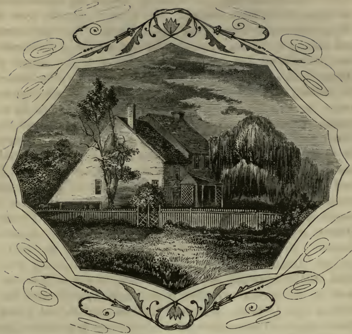
HEAD-QUARTERS AT BRANDYWINE.
