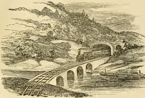
TUNNEL AND BRIDGE ABOVE PHENIXVILLE.
