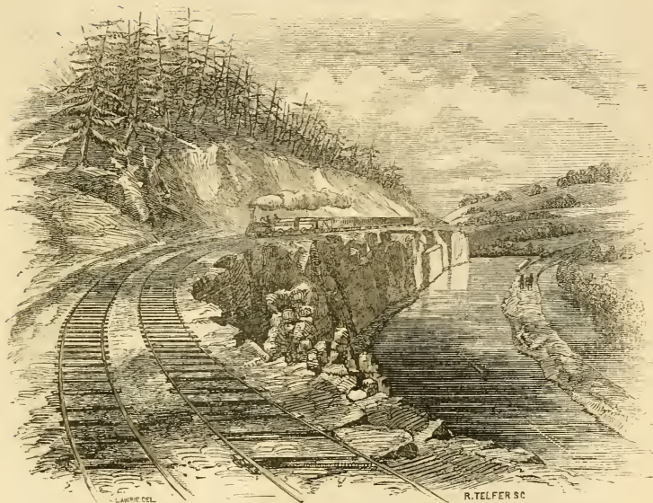
RAILROAD CURVATURE NEAR READING.
