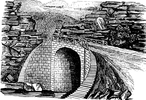
THE BIG VIADUCT, AND THE SHARP RIDGE ON THE WESTERN SIDE.
