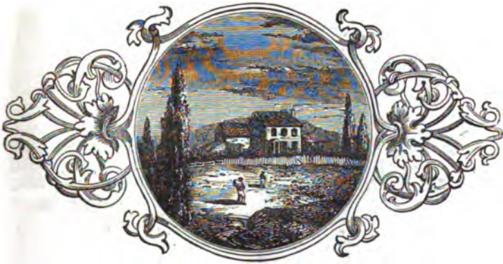
WASHINGTON'S QUARTERS AT VALLEY FORGE.
