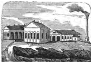
ENGINE-HOUSE AND WORKSHOPS.
