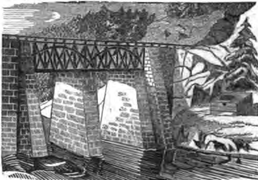
BRIDGE BELOW THE VIADUCT.
